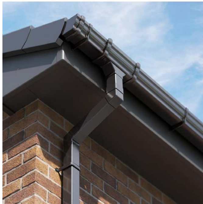
Fascias and Guttering - Black to match existing but changed to a modern square edged gutter
