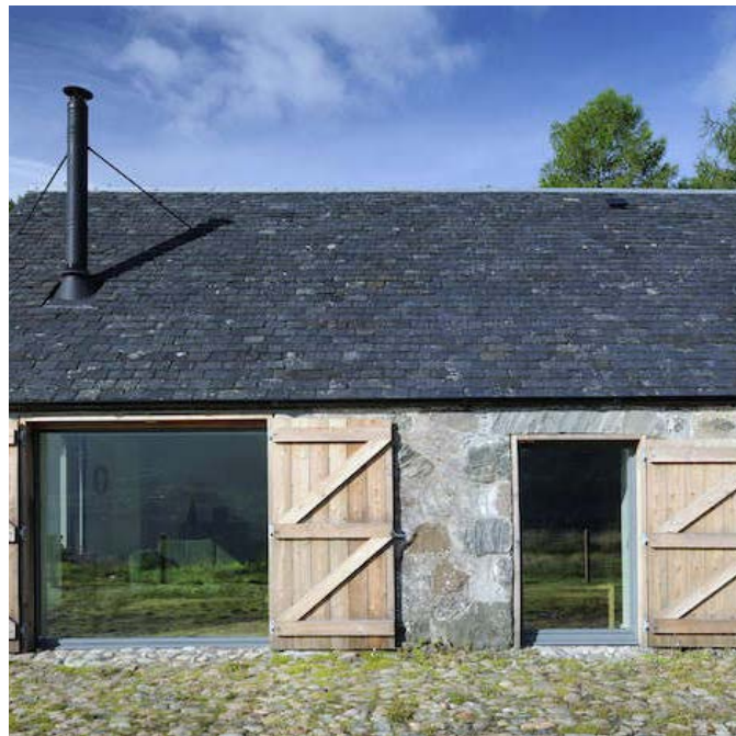
Slate Roof - Traditional slate roof
