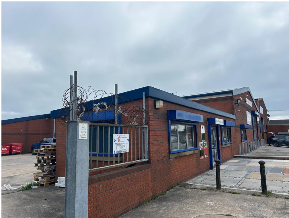
View From Lomax Street
