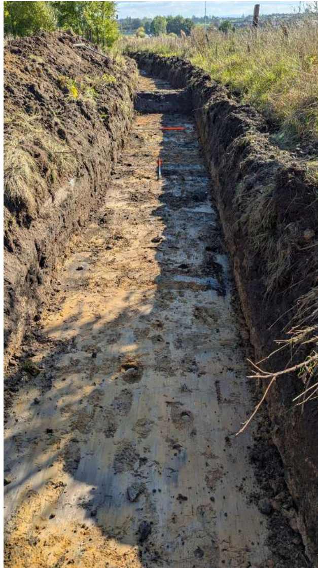
Plate 5- Trench 1, looking east
