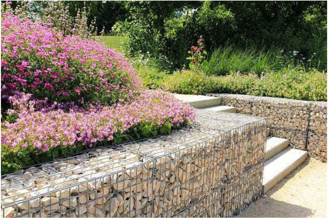
1M high gabion basket retaining walls
