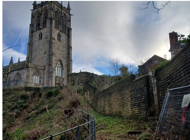
2.03 Before - Closer view of the Partnership House boundary wall, looking south towards Saint Chad's
