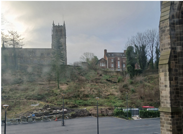
2.02 Before - View from Rochdale Town Hall looking south towards the Partnership House boundary wall
