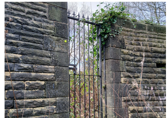
2.07 Before - Pedestrian gate proposed to be carefully removed and reinstated following construction works
