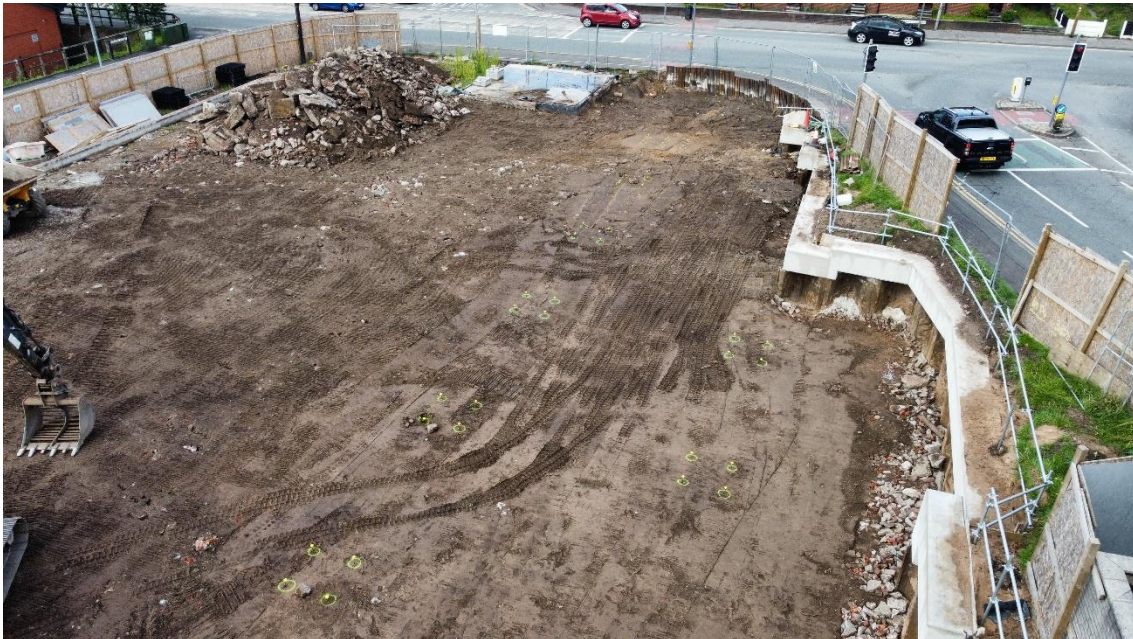
PLATE 3 – OVERSIZED HARDCORE STOCKPILE NORTHERN SECTOR OF THE SITE
