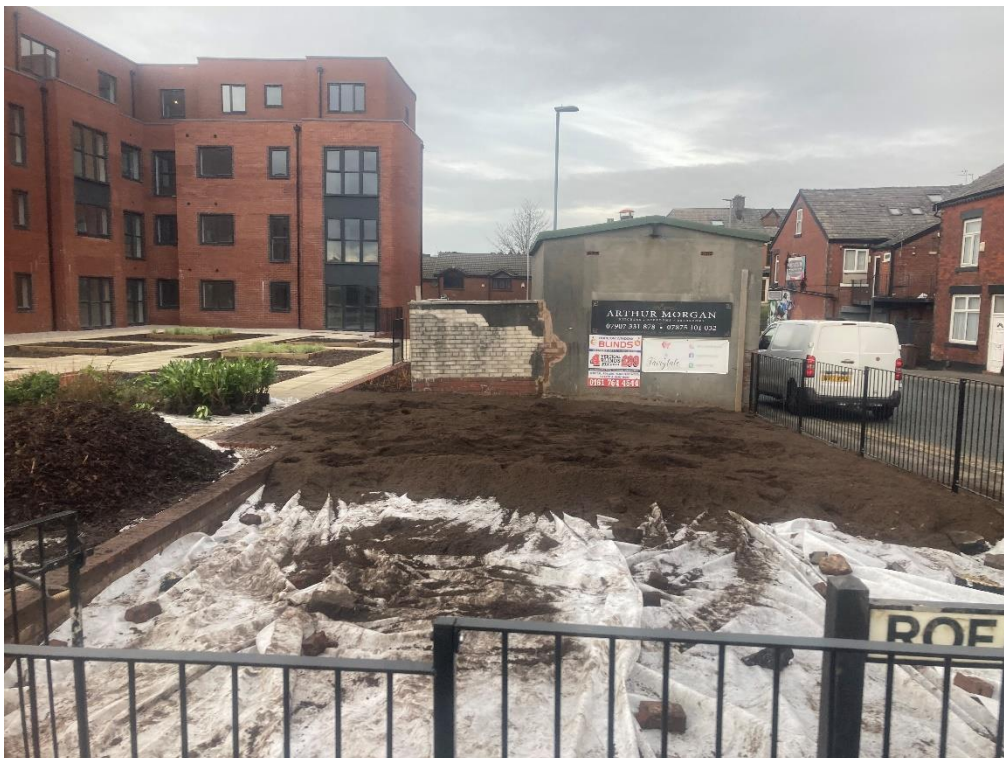
PLATE 4 – PLACEMENT MEMBRANE BELOW COVER SYSTEM
