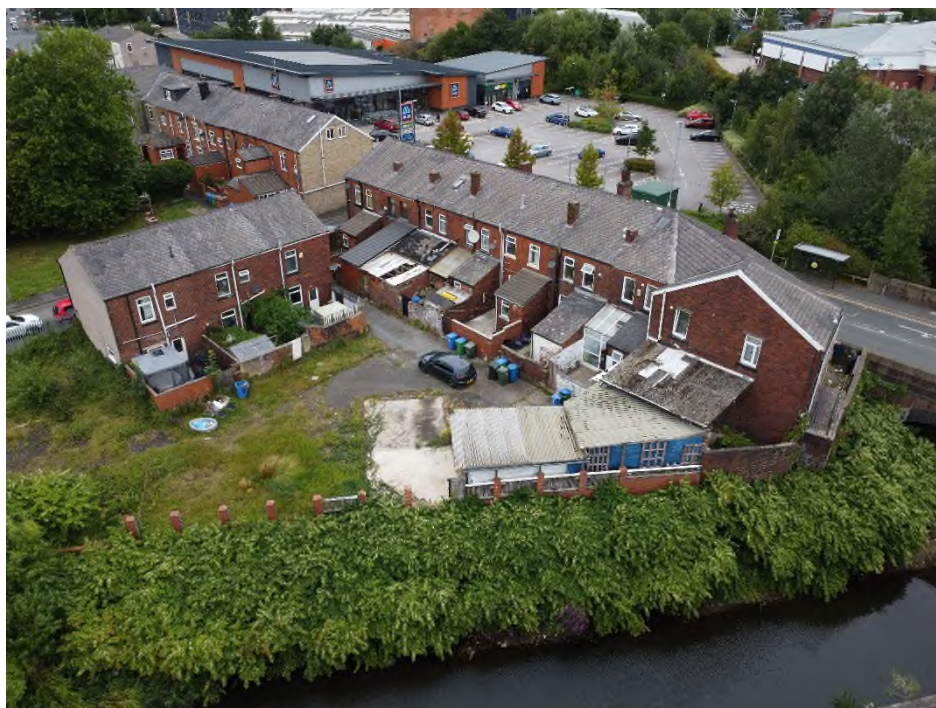
Photograph 4. Context view from rear
