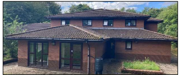
Leopold Court Hostel building: western aspects
