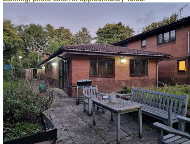
Photograph C: Photograph B: Projection on central north section of building; photo taken at approximately 19:30.
