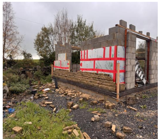
Existing Rear Elevation Photograph October 2025
