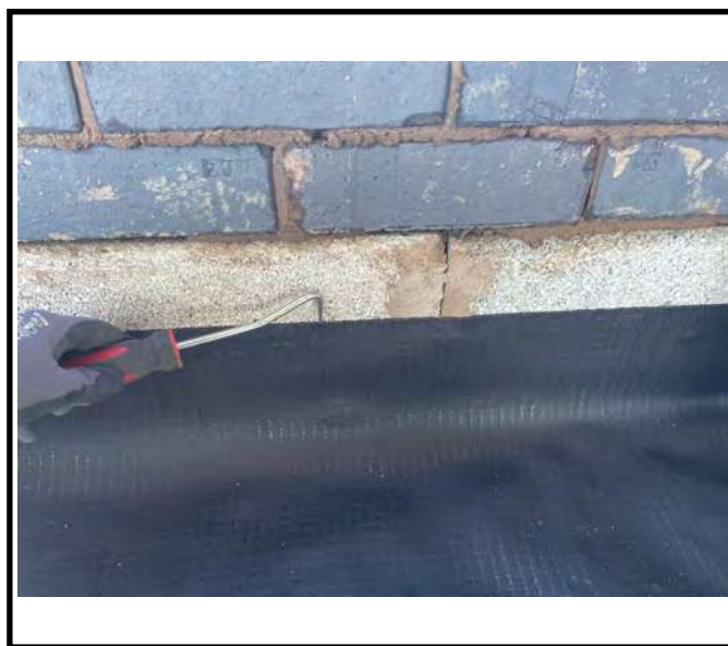
A mechanical point stress test being conducted upon the retrofit detailing around the perimeter.
