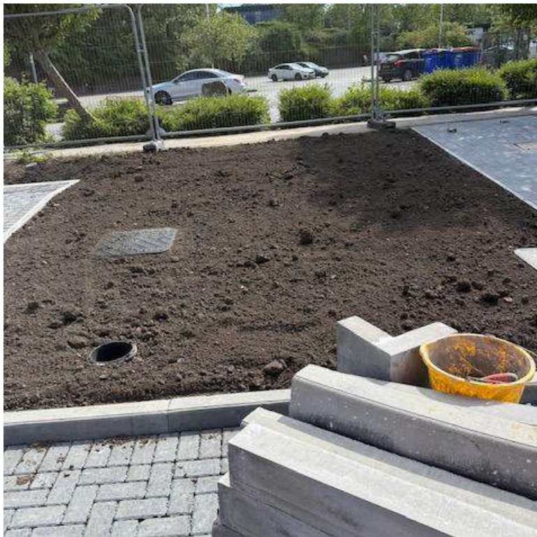
Photo provided by the Client of one of the landscaping planters with placed imported topsoil
