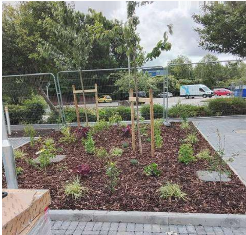
Photo provided by the Client of one of the landscaping planters showing it completed
