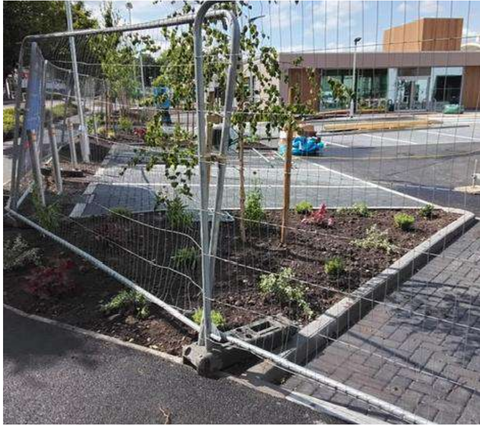
Photo provided by the Client of one of the landscaping planters showing it completed
