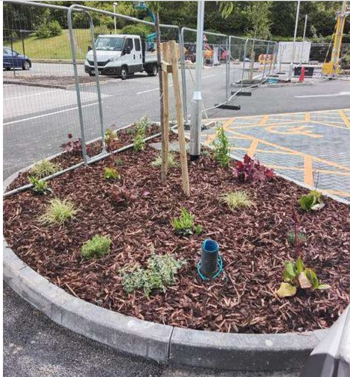
Photo provided by the Client of one of the landscaping planters showing it completed
