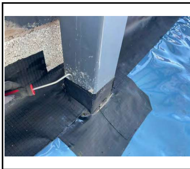
A mechanical point stress test being conducted upon a sealed steel stanchion.
