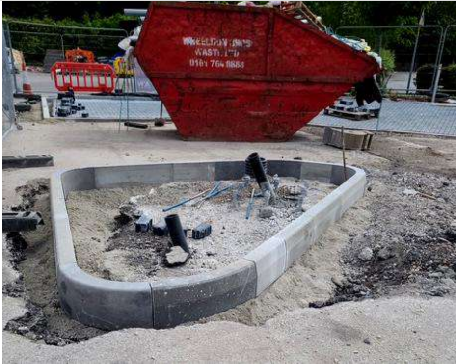
Photo provided by the Client of one of the landscaping planters pre-placement of topsoil
