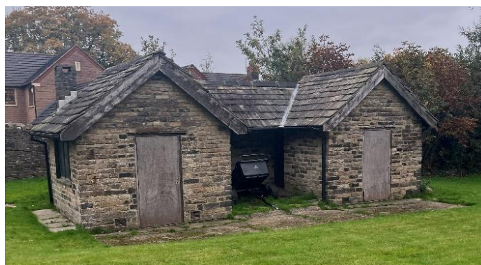
Fig 2.7 Exterior of stone buildings
