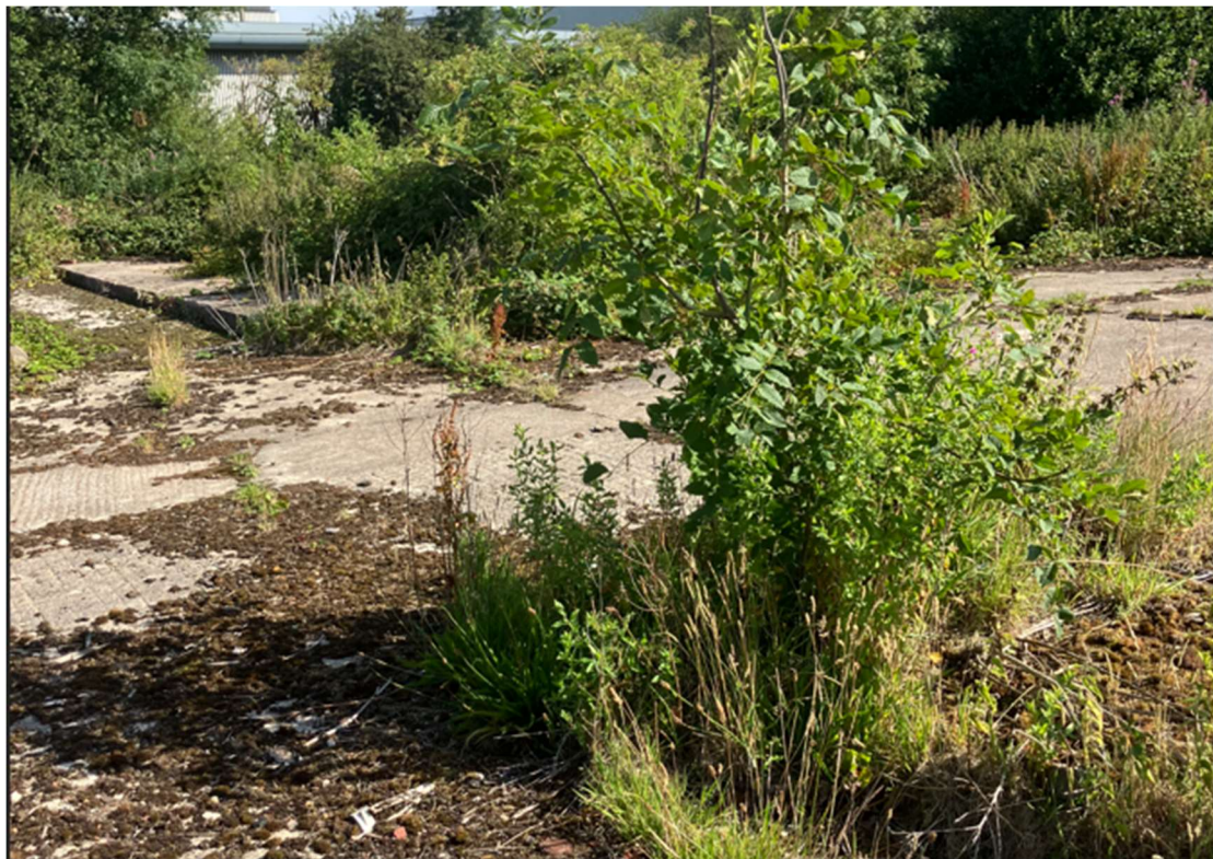
PLATE 3 – Remnant floor slabs at former Hares Hill Farm
