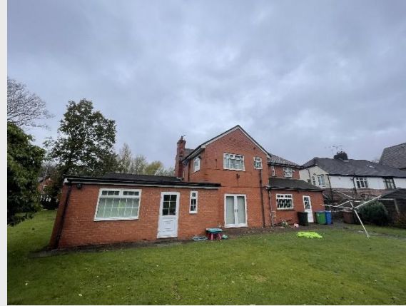
Photograph 2- Southern aspect of the building
