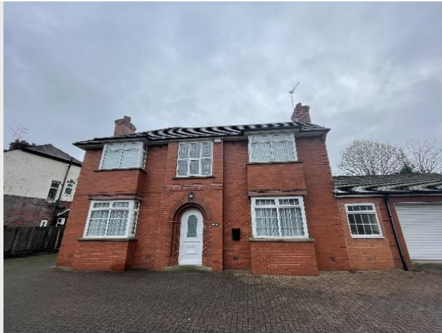
Photograph 1: Northern aspect of the building
