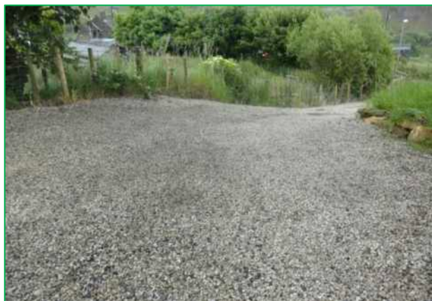
Access track; developed land sealed surface
