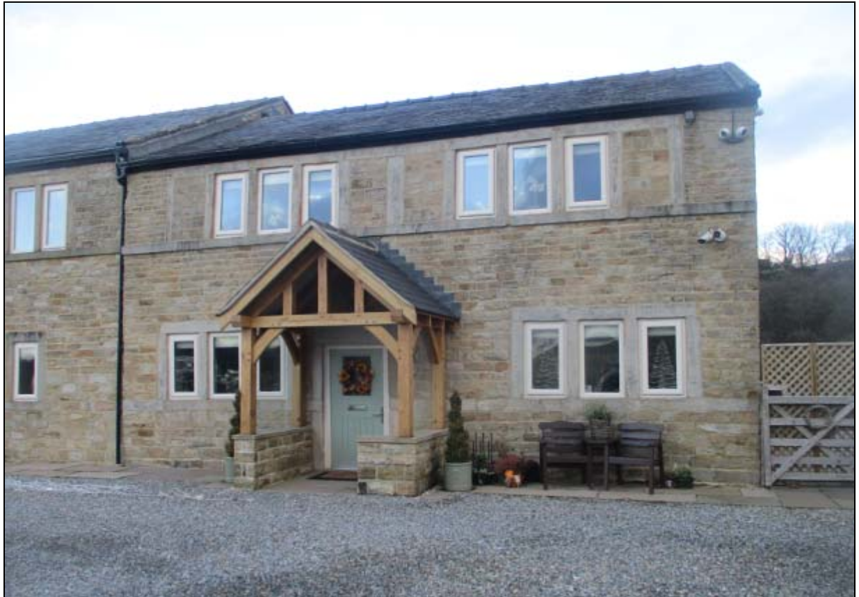
Front elevation of the house, with its former cottage doors and first floor weaver's window
