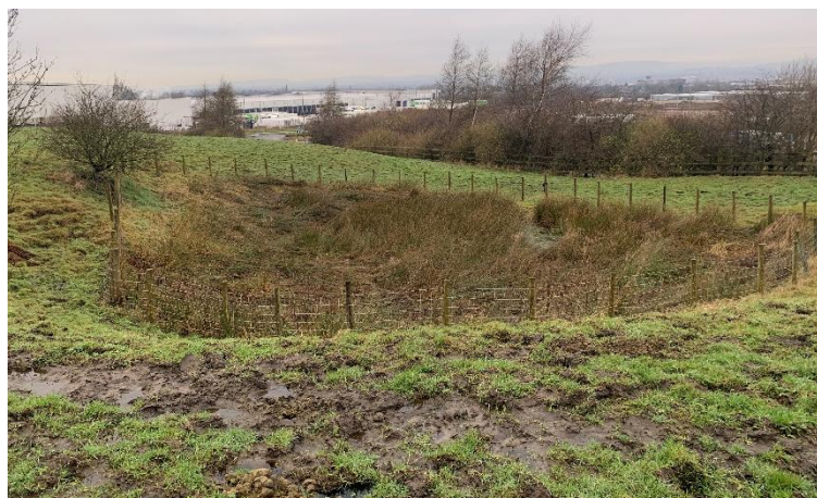
Figure 3: Photograph showing existing fence around the pond
