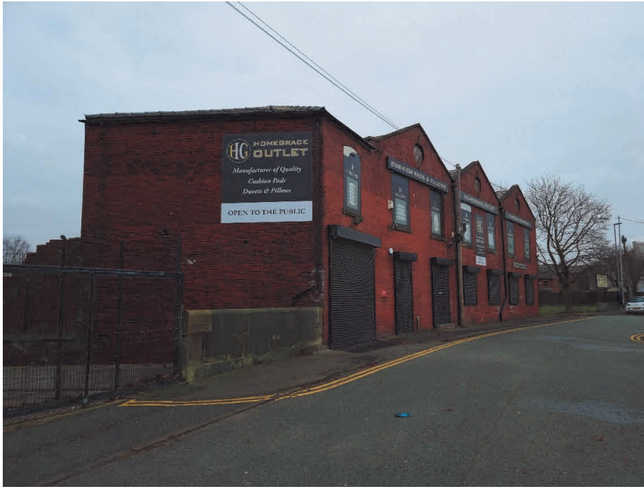
Photograph 1 – South East elevation of two storey mill, the proposed apartments are to be located on the first floor of this section of the building – elevation approximately 8.6m above the Sudden Brook
