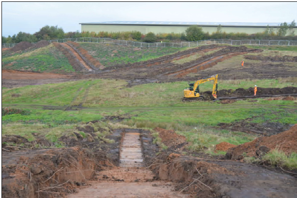
Plate 2. General view of site, looking north
