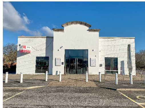
02 View of the front elevation South-west.
