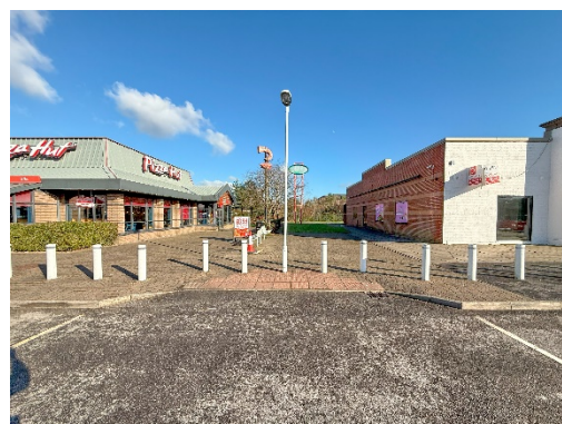
A View of former Pink Drips unit and Pizza Hut from the carpark.
