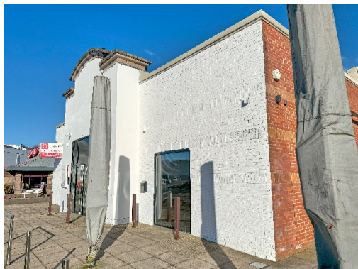
01 View from car park.
