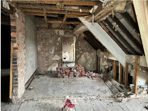
Masonry stored at second floor
