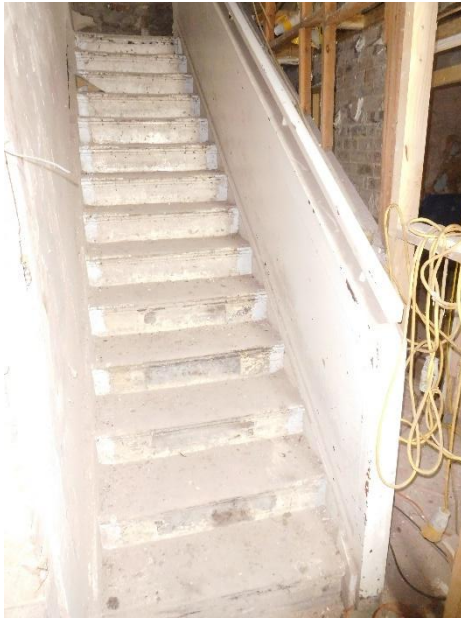
Stair from ground up to half landing
