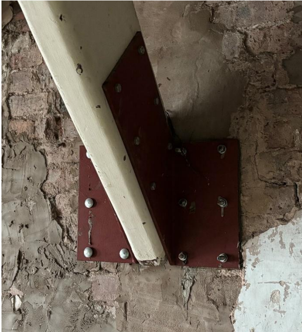
Valley bracket connection to wall
