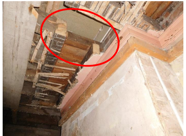
Trimmers cut in front of chimney breast
