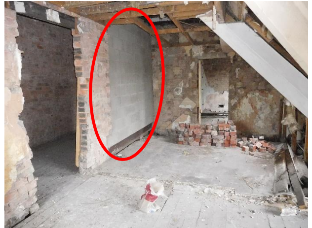
Blockwork wall built on steel beam
