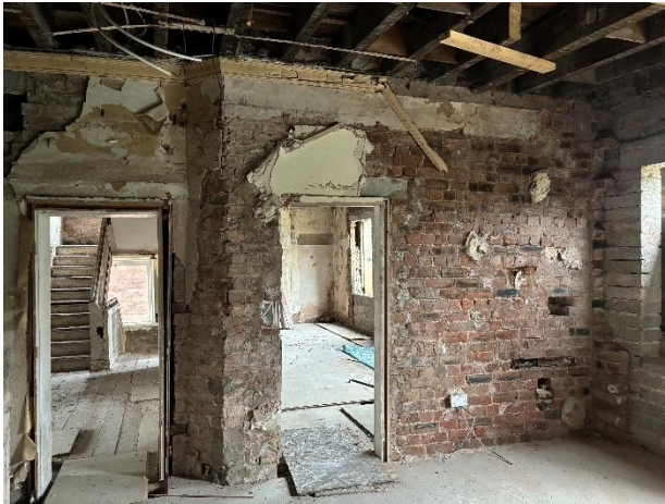
View towards stairwell from rear righthand room
