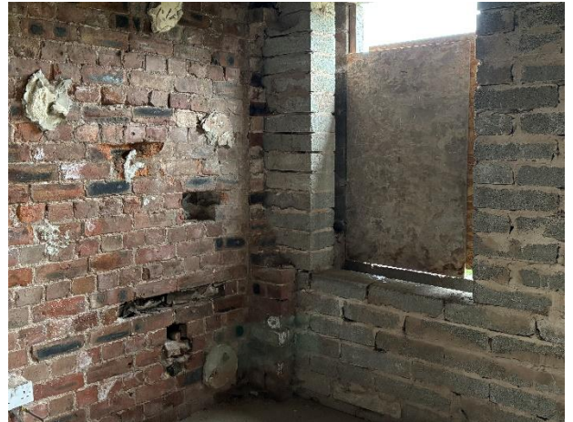
Junction of rear and internal walls
