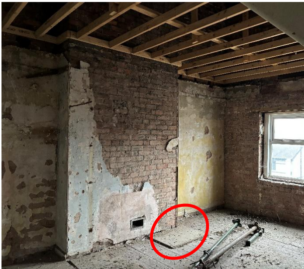
Boarding over cut floor trimmer
