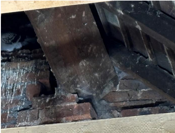
Upper purlin bearing into front gable
