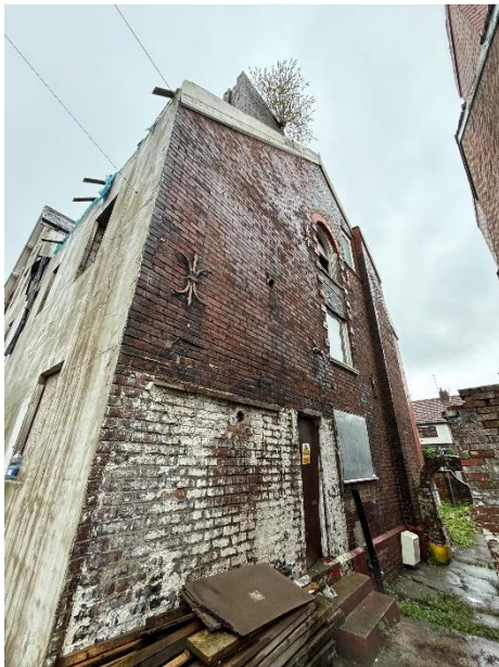
Lefthand gable viewed from rear
