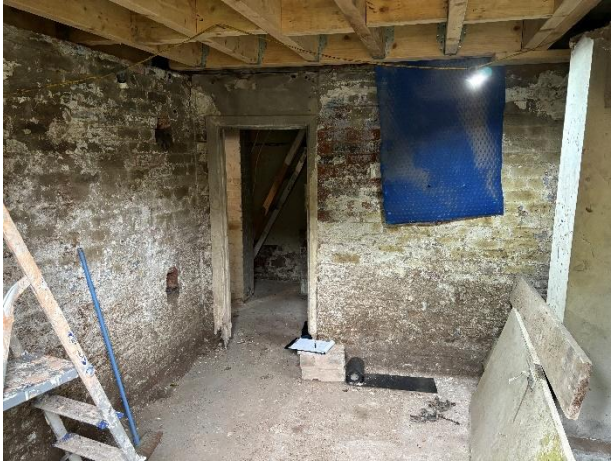
View towards front in rear lefthand room
