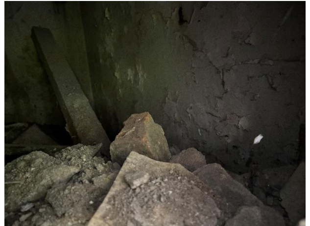
View into void behind block wall
