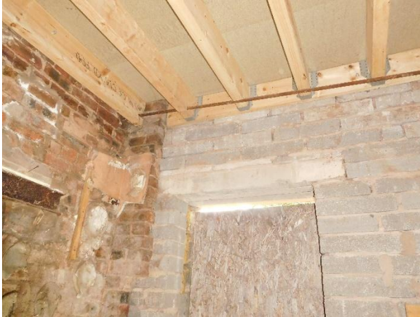
Junction of original dividing wall and new rear wall
