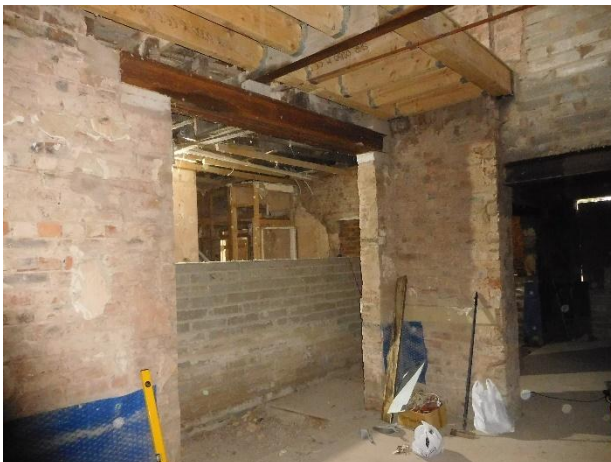
Opening in wall between hallway and front righthand room
