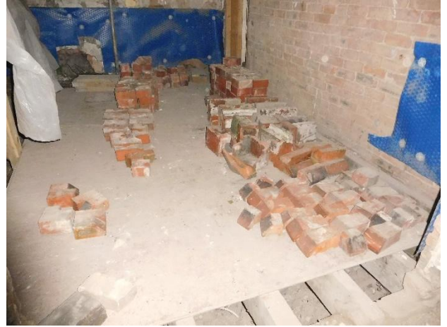
Masonry from bay window stored on floor
