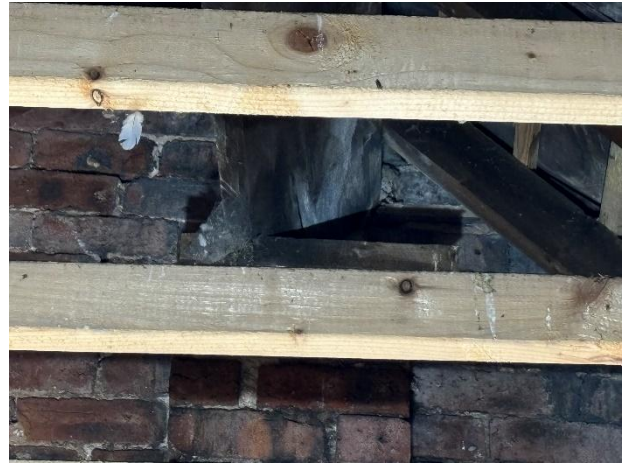
Lower purlin bearing into front gable
