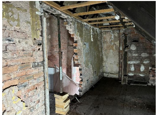
Opening between rear room and stairwell
