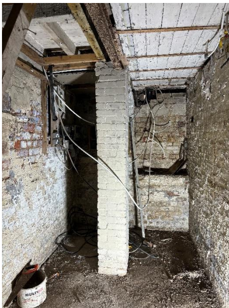
View towards left below stairwell
