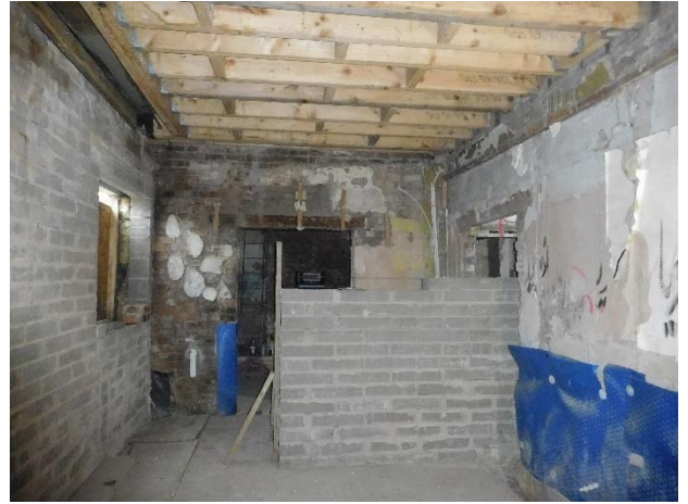
Rear end of dividing wall in rear room
