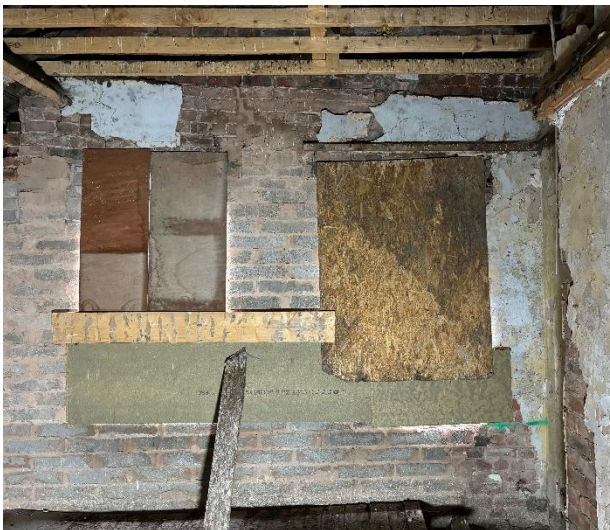
Rear wall constructed in blockwork up to window head. Note, sloping bedjoints in original masonry above window
