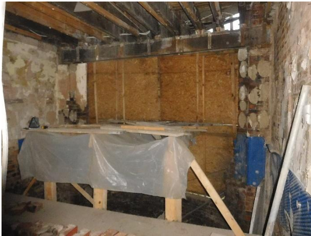
Front elevation where bay has been dismantled
