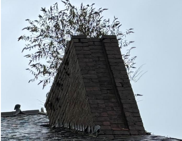
Rear lefthand chimney stack
