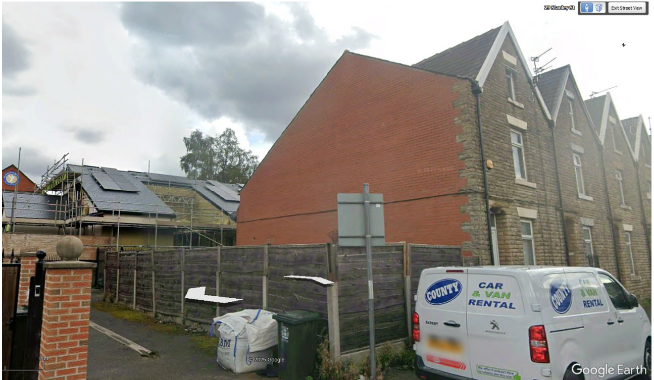
Google Earth Streetview Image of Development Plot & Gable of Existing Terrace
