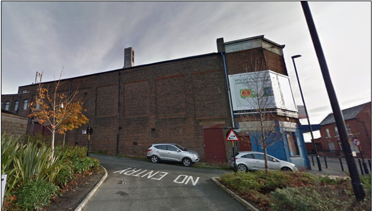
Figure 1: Streetview of the subject site.
