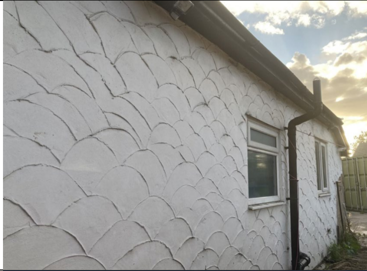
Photograph 4- Eastern elevation showing the render finish.
