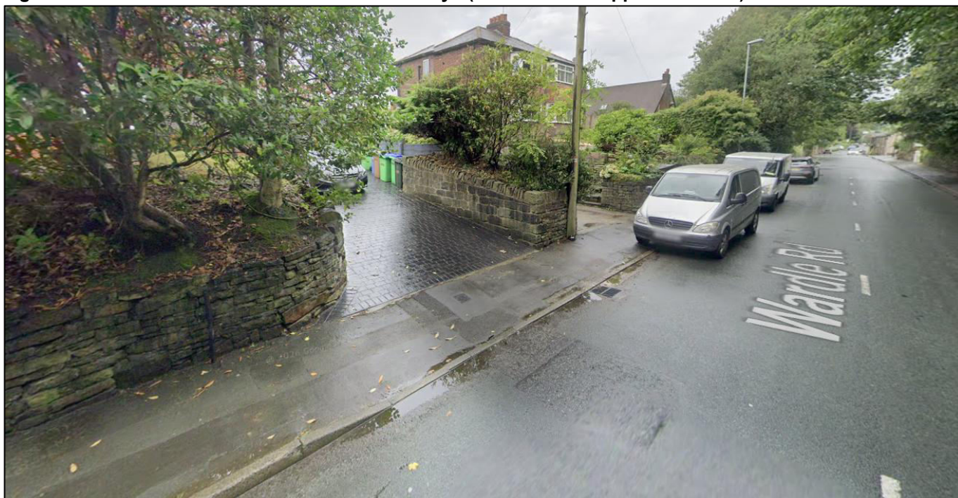
Figure 6: View of 191 & 191 Wardle Road Driveways (50m South of Application Site)
