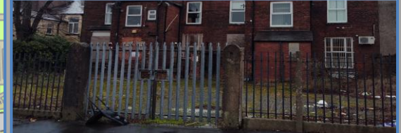
A view of the rear elevation and rear boundary fencing and gates to number 153-195
