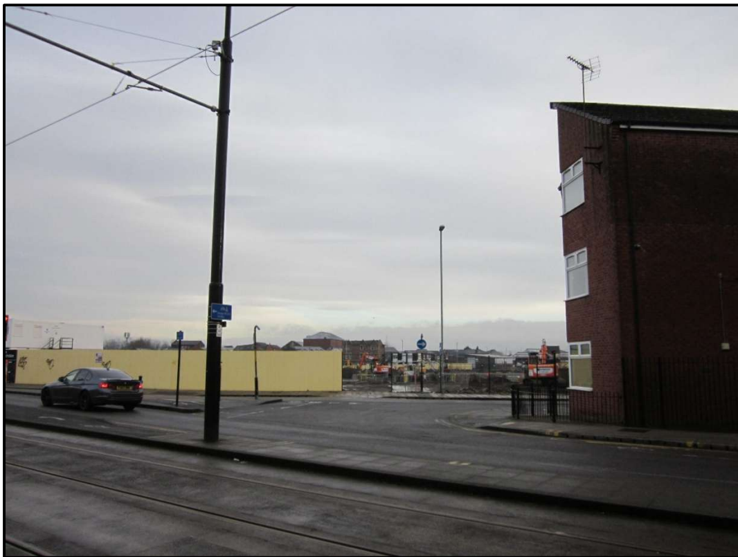
Photograph 3. Site of the proposed new Rochdale Sixth Form and Hopwood Hall College (looking North East)
