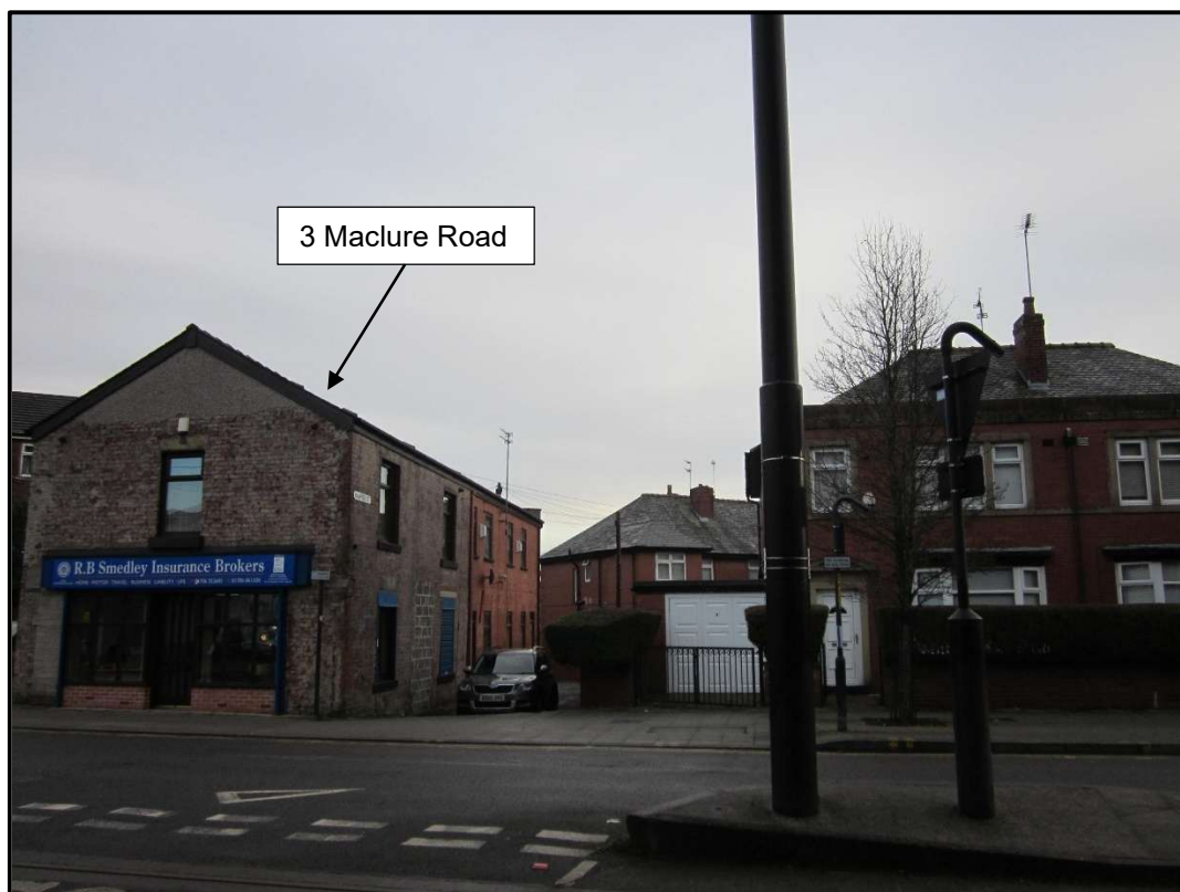
Photograph 1. Existing commercial office building at 3 Maclure Road, Rochdale (looking East)
