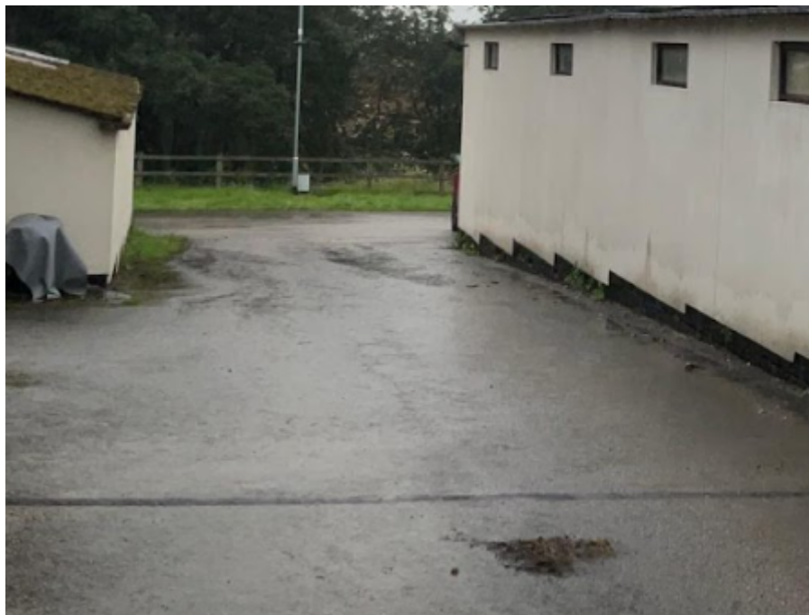
Photograph 1 - u1b Developed land - sealed surface (concrete yard)
