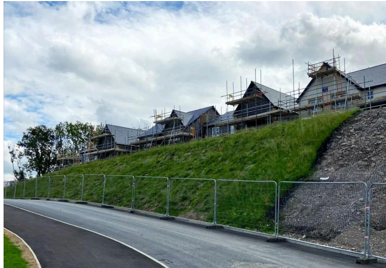
Engineered Reinforced Slope
