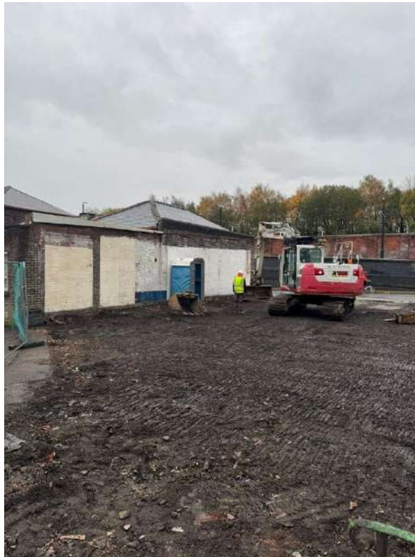
Photograph 3 – West of site and adjacent commercial building
