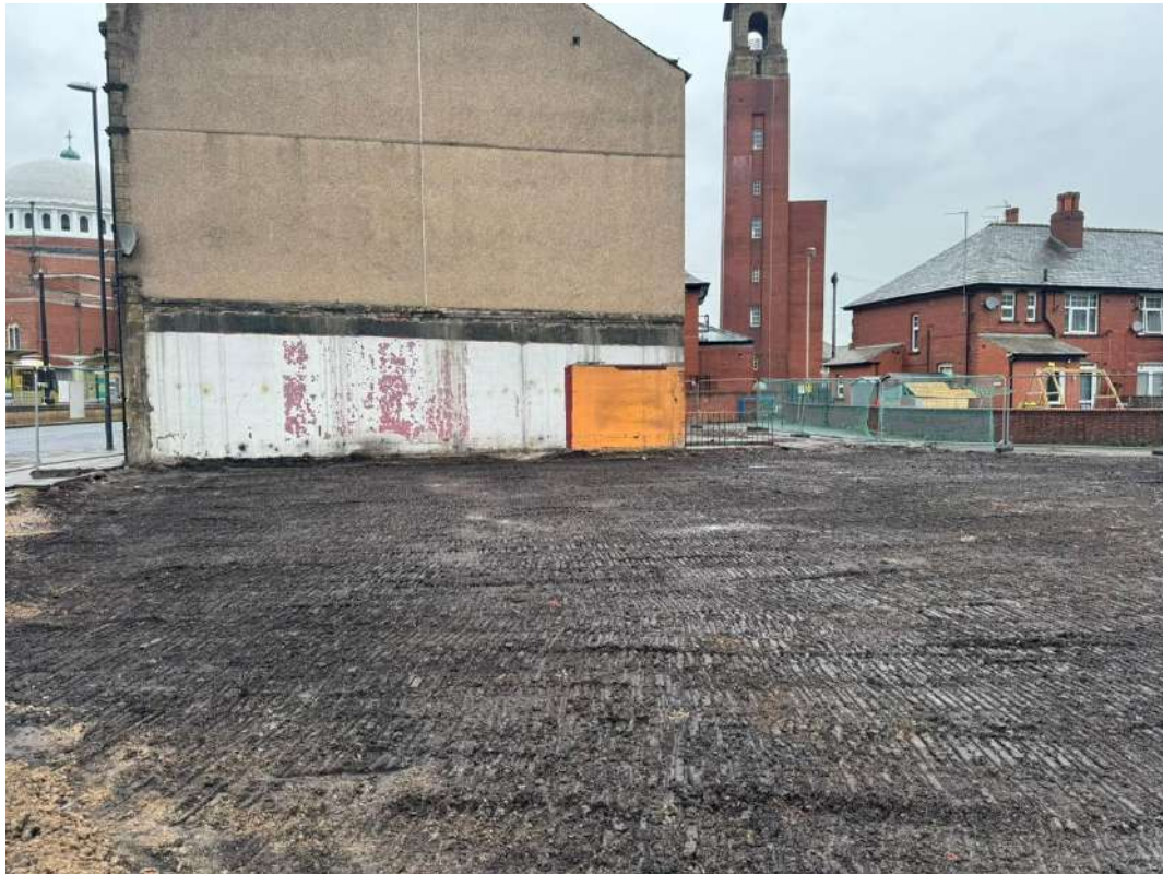
Photograph 1 – Building to be retained in the north of the site
