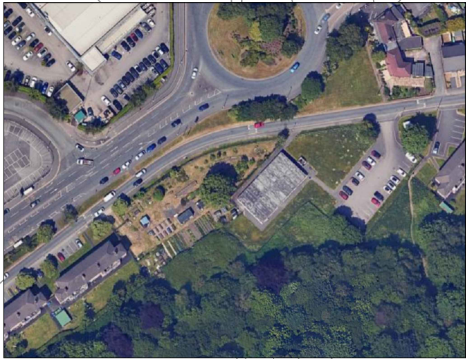
NORTH SOUTH AERIAL VIEW
