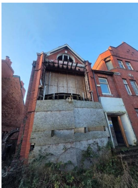
37 Rochdale Road Front View
