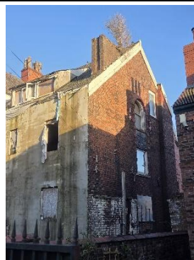
Lefthand gable viewed from rear
