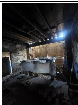
Front elevation showing dismantled bay
