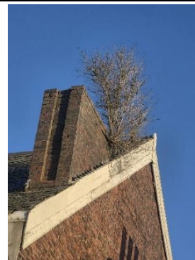
Rear lefthand chimney stack
