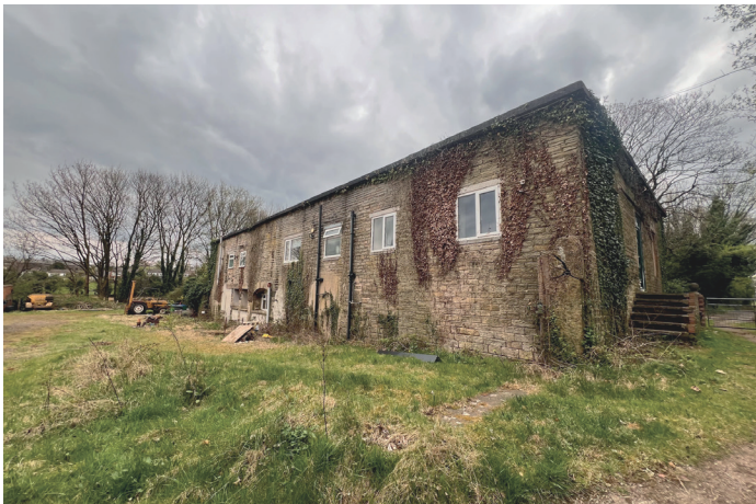
Rear Elevation of the Existing Calliards Mill
