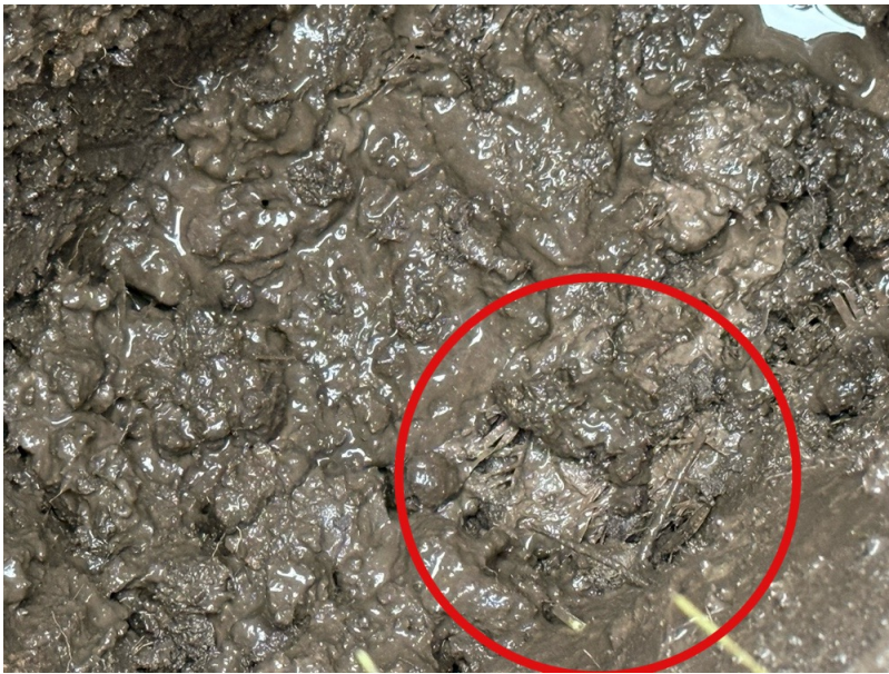
Photo 12 Plot 60 geotextile at base of capping layer
