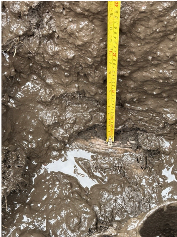
Photo 7 Plot 57 after water bailed out showing geotextile membrane beneath capping layer
