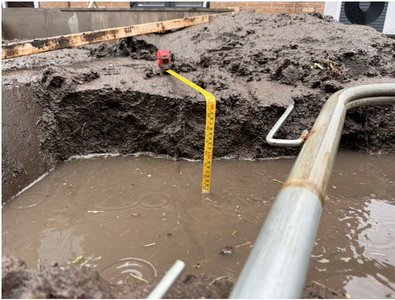
Photo 3 600mm capping present in plot 56
