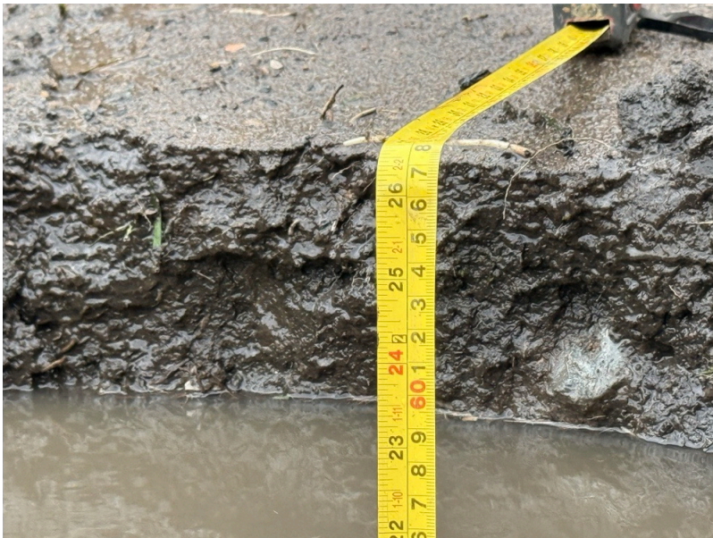
Photo 6 Plot 57 600mm capping before water bailed out
