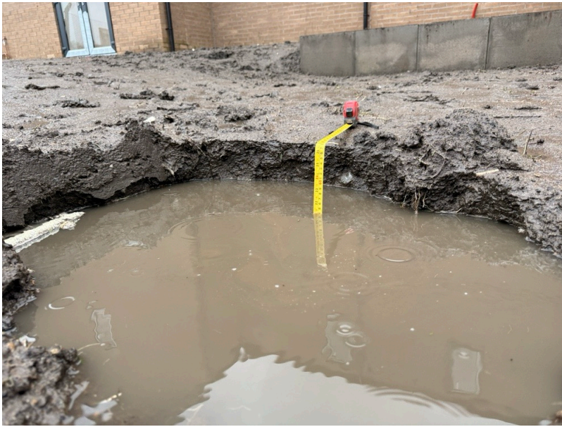
Photo 5 Plot 57 600mm capping before water bailed out
