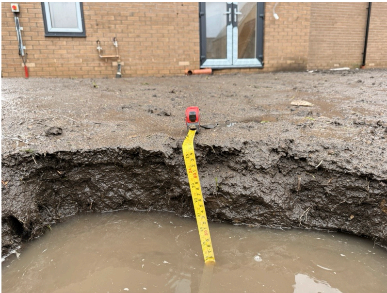
Photo 8 Plot 58 600mm capping layer
