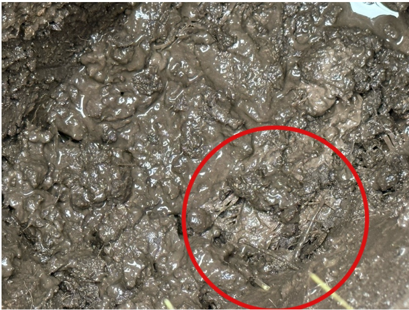
Photo 12 Plot 60 geotextile at base of capping layer
