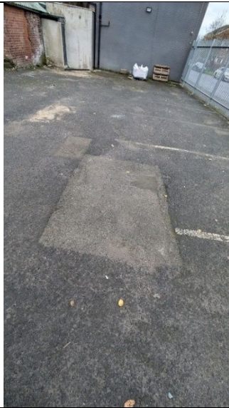
Photograph 3: Repair to car park. Former public house building visible.
