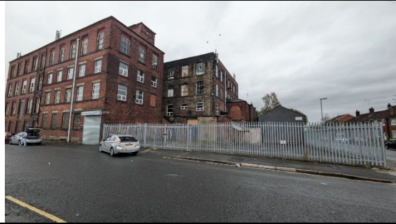
Photograph 1: View SW of site from the NW. Behind palisade fencing (L-R) substation, former engine house and former public house building. .
