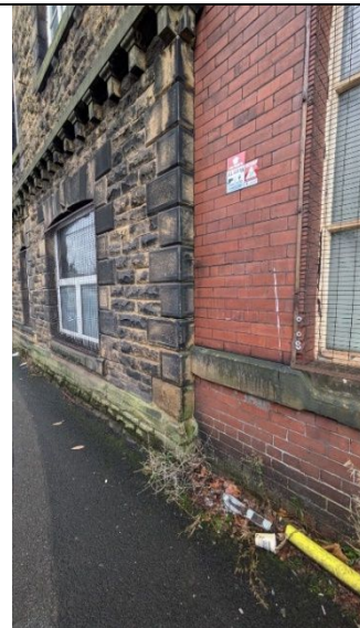
Photograph 6: View SW of eastern elevation from Duke Street. No evidence of cellar / lightwells below stone fronted section .
