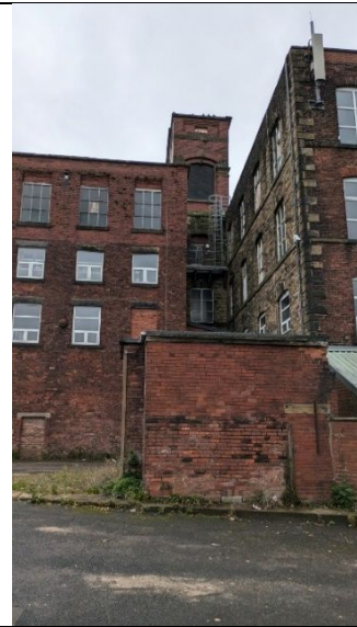
Photograph 4: View of western elevation. Shaft / lift feature which is higher than the 4 th storey is visible centre of photo.
