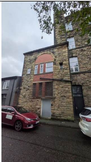
Photograph 5: View N of the former engine house (proposed entrance area) from Queen Street. Former public house to left of photo. Flue visible.
