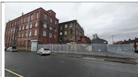
Photograph 1: View SW of site from the NW. Behind palisade fencing (L-R) substation, former engine house and former public house building. .
