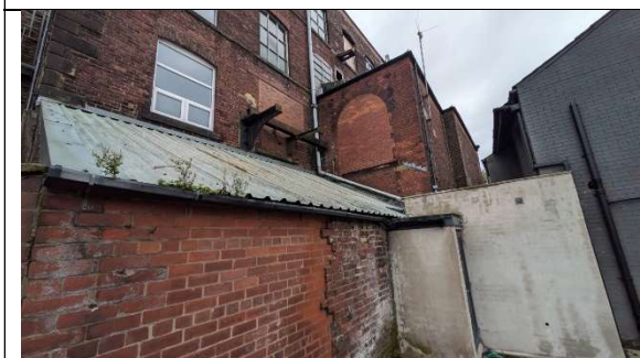
Photograph 5: View S showing roof drainage to the north of the former engine house.
