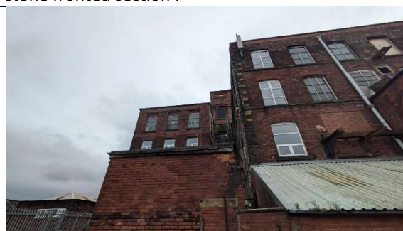
Photograph 6: View of eastern elevation. Roof drainage visible to right of photograph.
