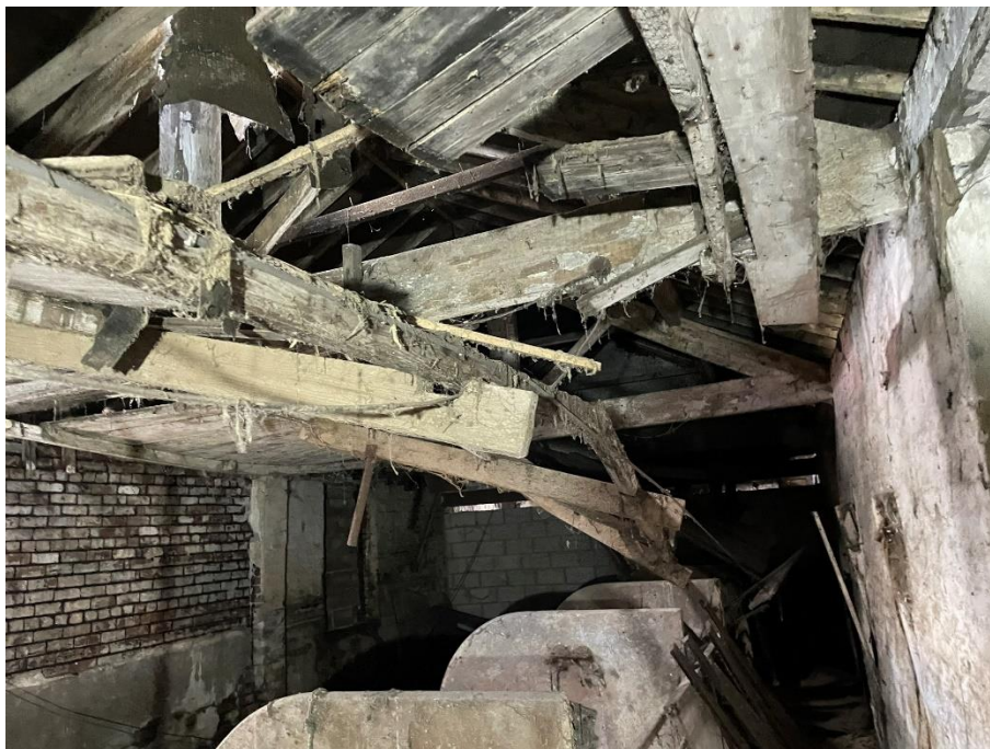
Photo 14 Barn Single Storey Ceiling
