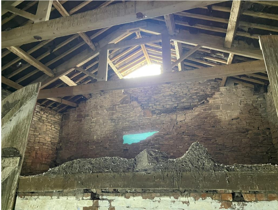
Photo 11 Barn Two Storey Section Showing West Elevation Gable End
