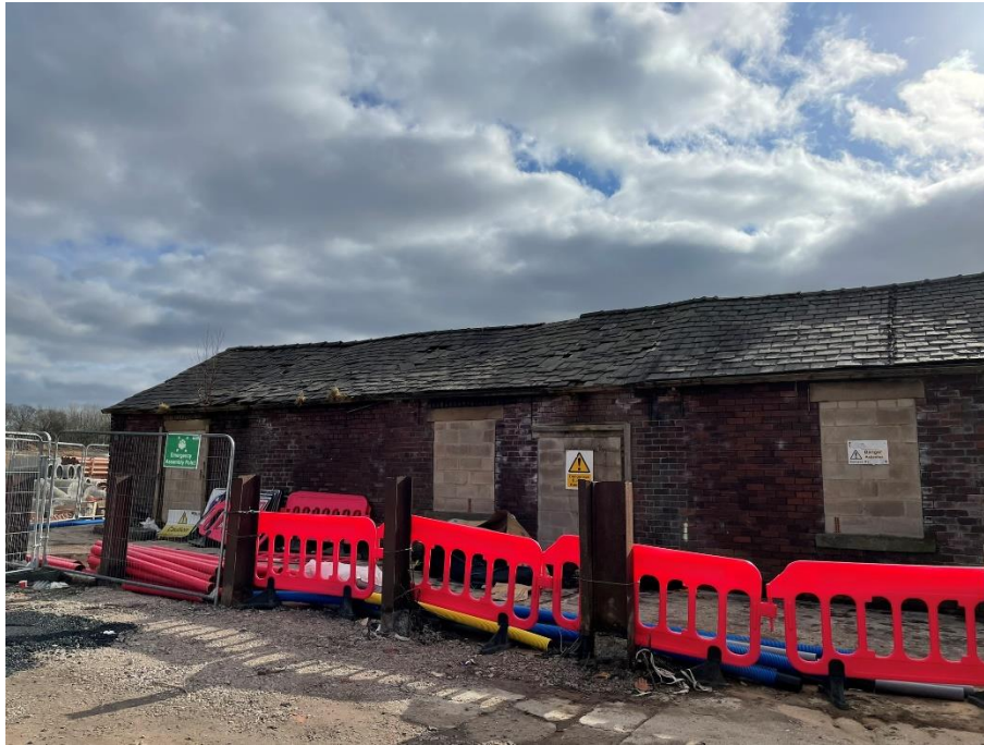
Photo 4 Barn North Elevation Showing Single Storey Section
