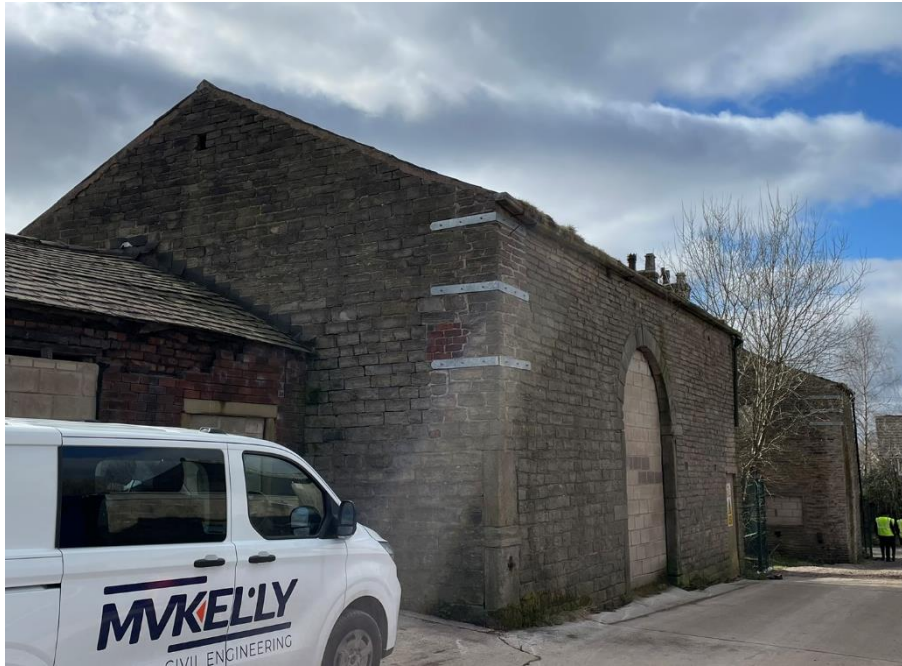
Photo 10 Barn North Elevation
