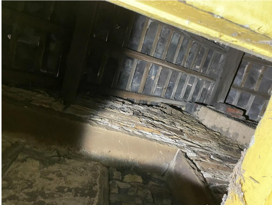
Photo 22 Farmhouse Roof Structure
