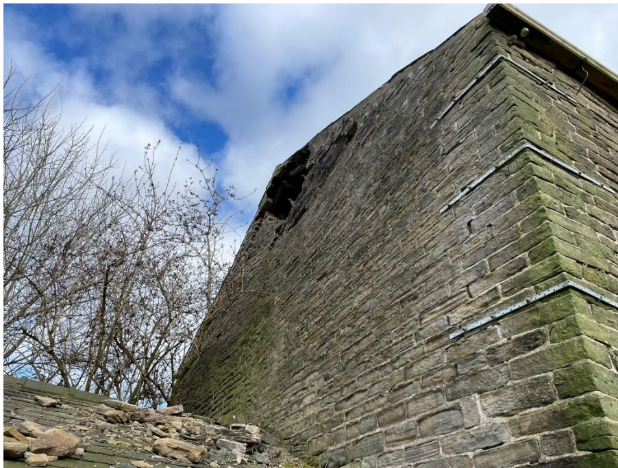
Photo 9 Barn West Elevation on Gable End
