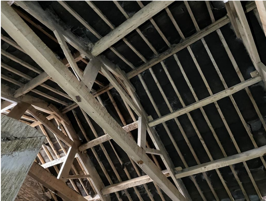
Photo 12 Barn Two Storey Section Showing Roof Structure
