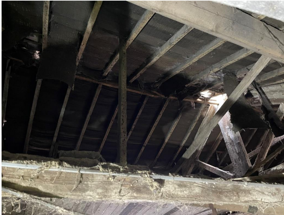
Photo 13 Barn Single Storey Roof Structure
