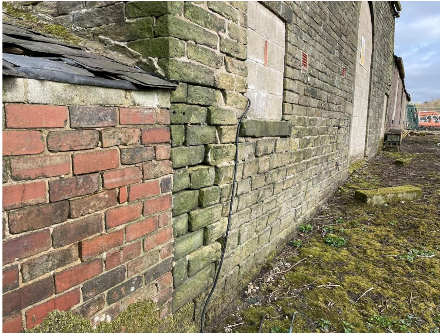
Photo 6 Barn South Elevation
