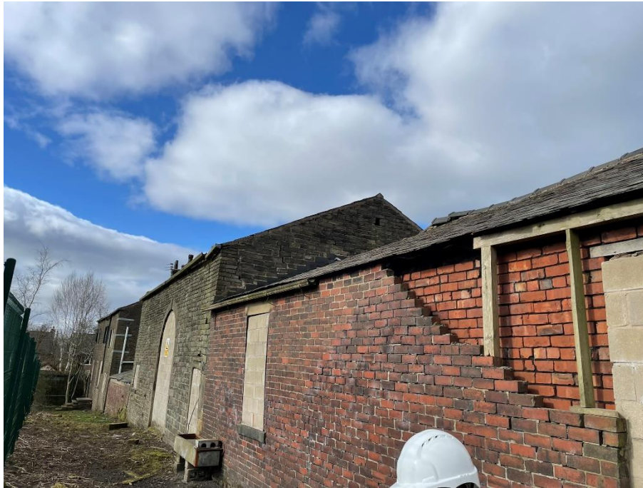
Photo 8 Barn South Elevation Between Single & Two Storey
