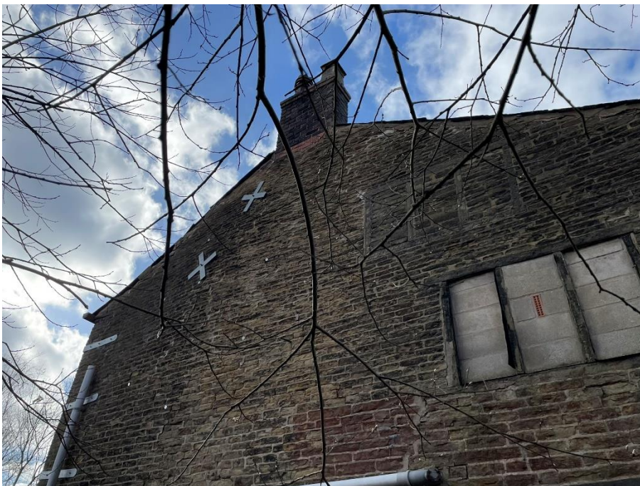
Photo 16 Farmhouse East Elevation on Gable End
