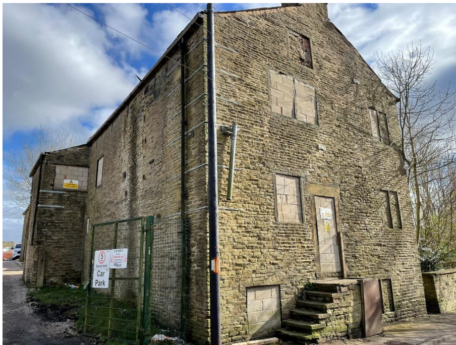
Photo 18 Farmhouse West Elevation on Gable End
