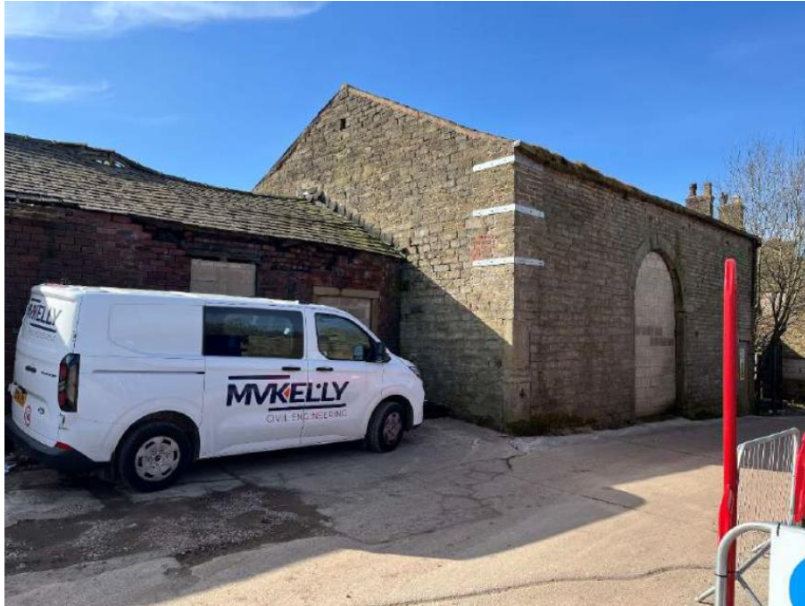
Photo 3 Barn North Elevation Showing Two-storey Section
