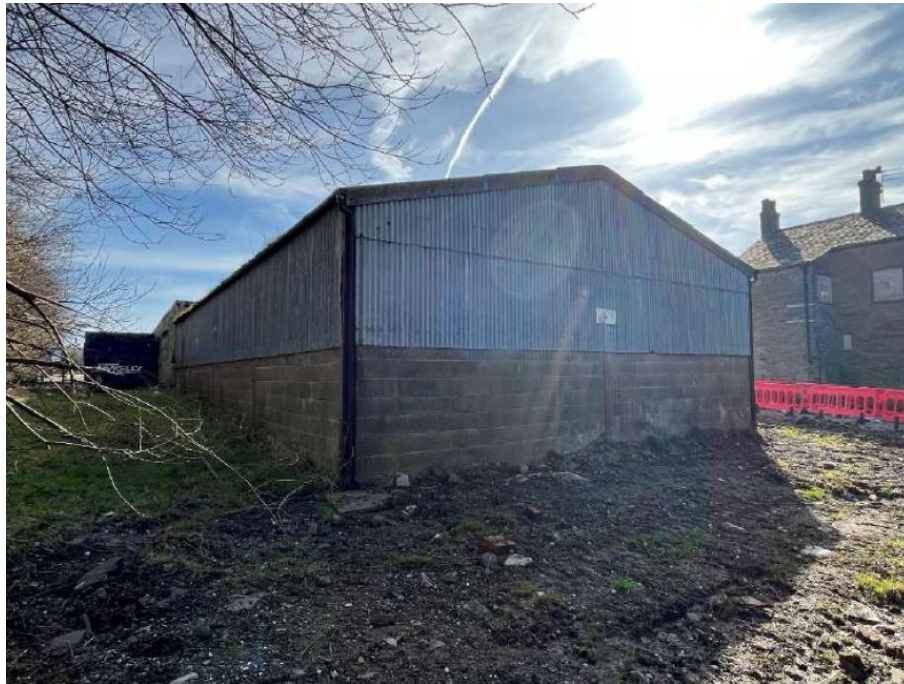
Photo 1 Out-building North-West Elevation
