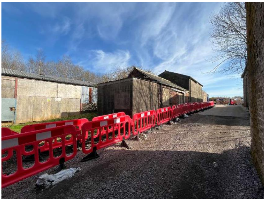
Photo 2 Out-building South-West Elevation
