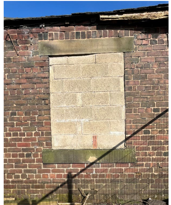
Figure 11 – Opening within former outbuilding, surrounds intended for reuse within the development
