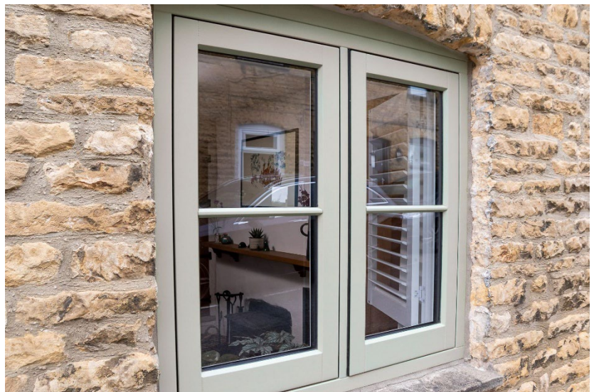
Figure 06 – Example of a timber window within a stone wall
