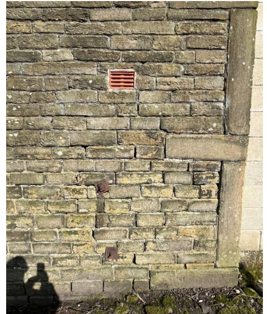
Figure 01 – Existing natural facing stone
