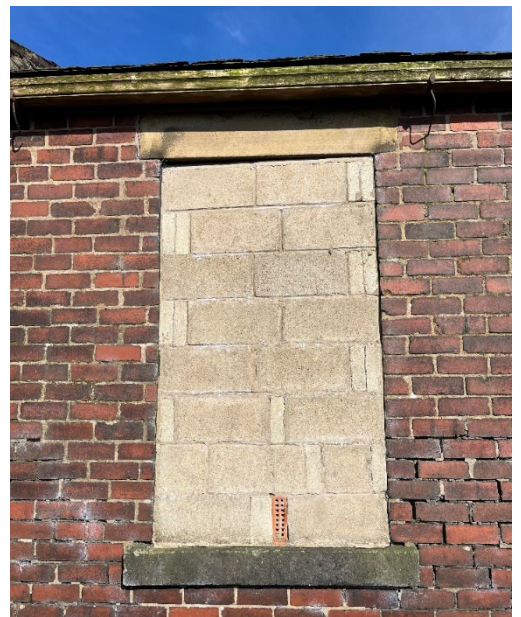
Figure 02 – Existing red facing brick
