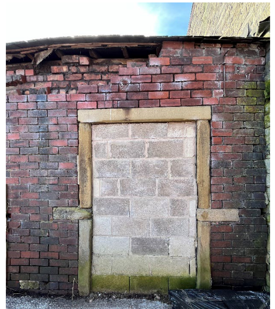
Figure 12 – Opening within former outbuilding, surrounds to be reused to form main entrance into the converted barn within the new extension
