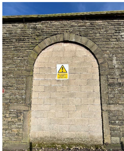
Figure 10 – Existing stone surrounds to arched opening within the barn
