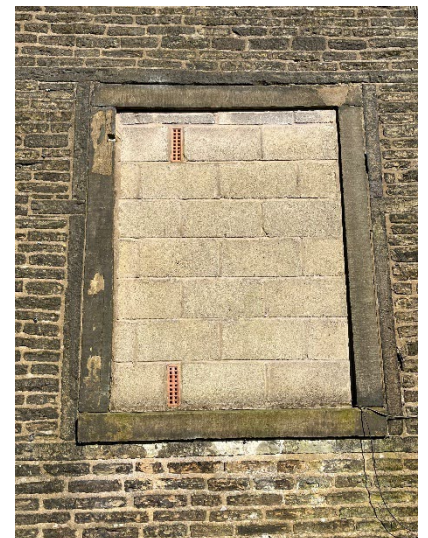
Figure 09 – Existing stone surrounds
