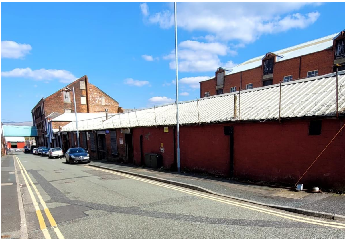
Fig 1. Image showing existing industrial building from Hill Street
