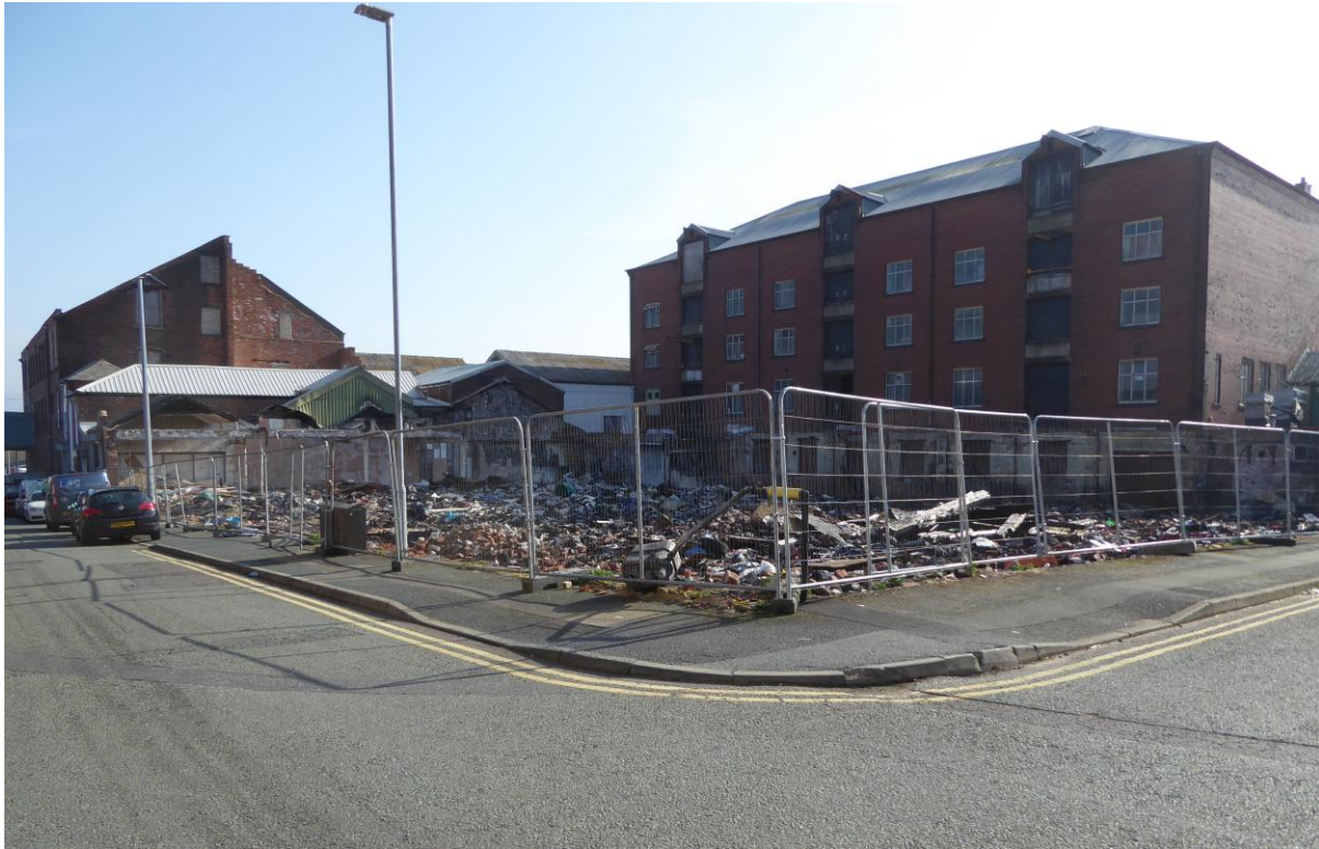
Fig 3. Image showing extent of existing site from corner of Hill Steet and Summer Street
