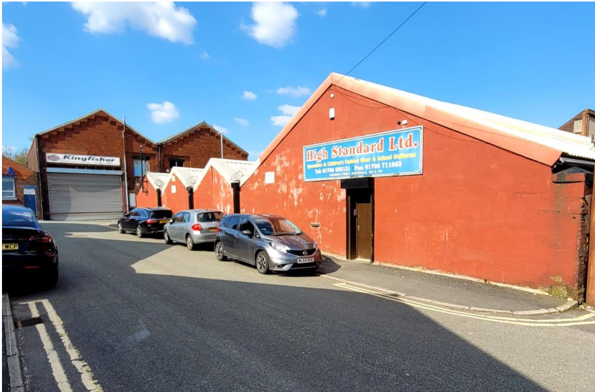
Fig 2. Image showing existing industrial building from Summer Street
