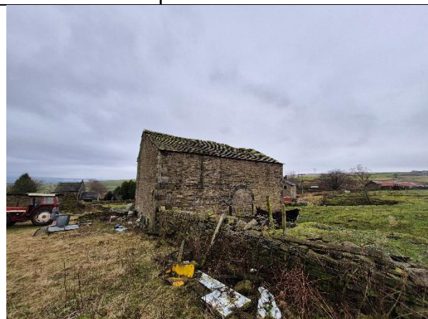
Photo 11: Northern facing side of building 1.
