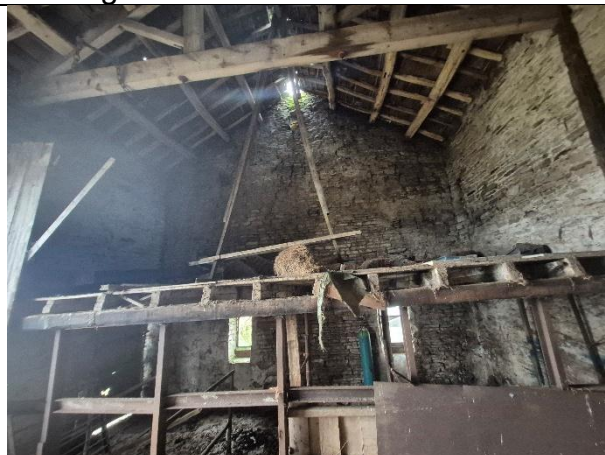
Photo 18: View of western side of building 1.
