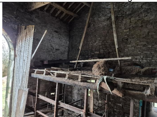
Photo 21: Western facing view of second story.
