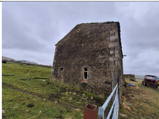
Photo 2: West facing side of building 1.
