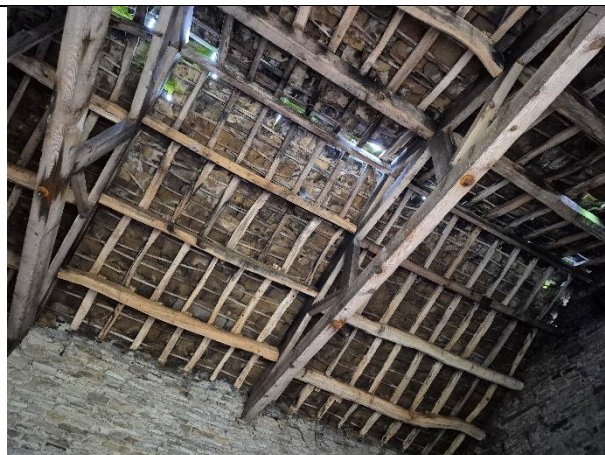
Photo 14: Inside view of tiled roof of building 1.
