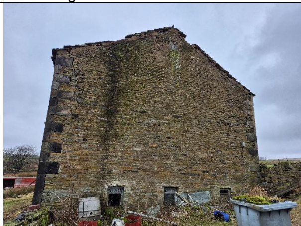
Photo 6: East facing side of building 1.
