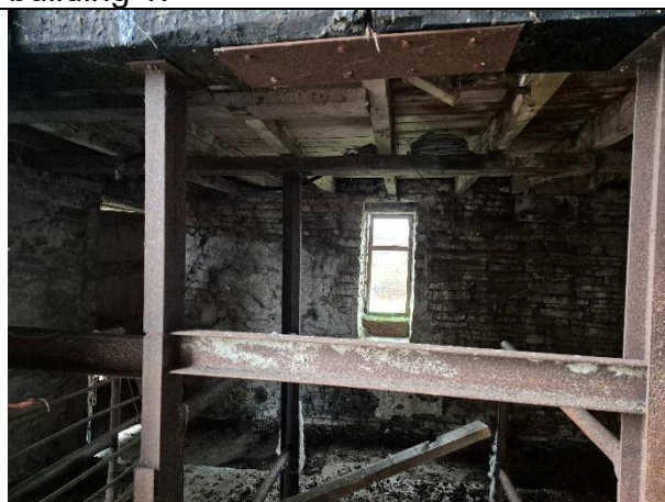
Photo 16: Lower storey facing east inside building 1.
