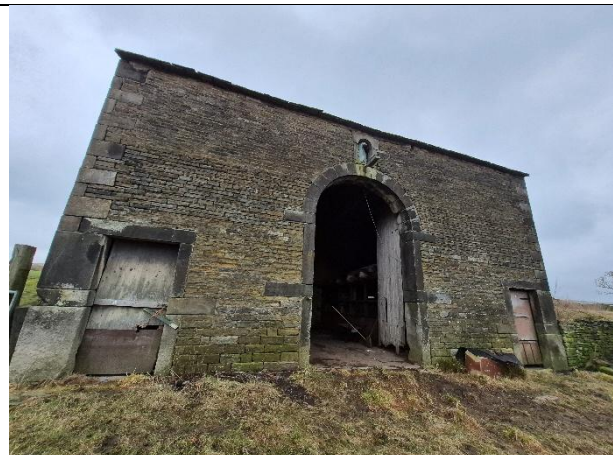
Photo 1: South facing side of building 1.
