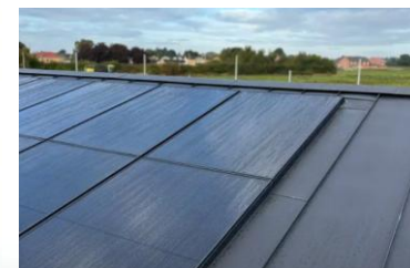
Integrated solar panels with metal surround and flashing
