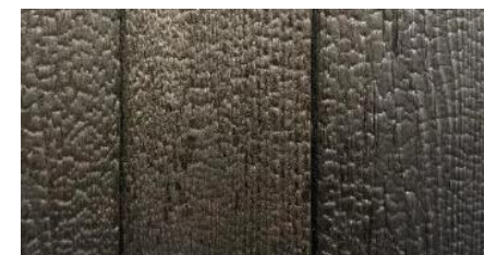
Charred Timber Cladding
