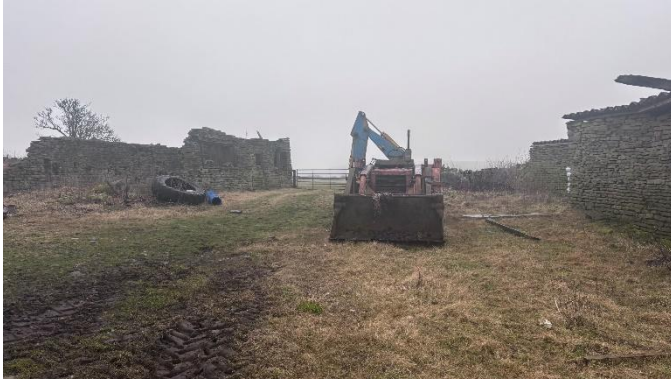
Plate 5 View showing the eastern site boundary
