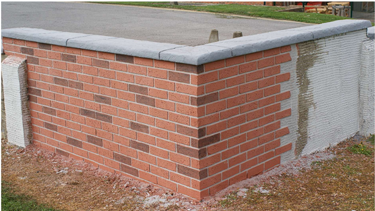
Figure 2: Brick effect render on retaining wall showing clear difference of before the render being applied and after. (Google Images)
