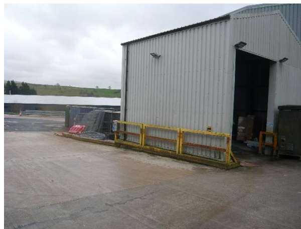
Photo 4: Habitat 2: Buildings and Habitat 3: Hardstanding
