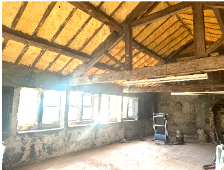
Photograph 5- Second-floor Attic Room with spray foam insulation visible
