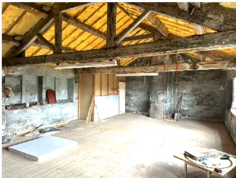
Photograph 6- Second-floor Attic Room with spray foam insulation visible
