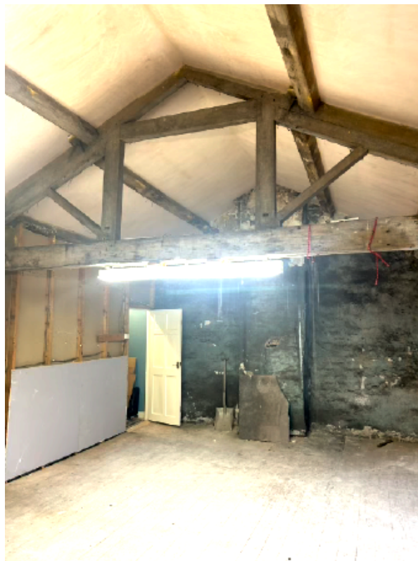
Photograph 4- Existing Second-floor Attic Room
