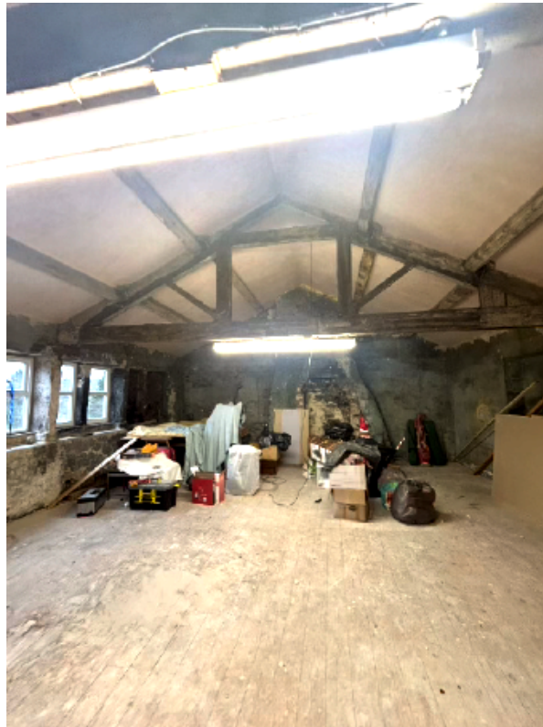
Photograph 3- Existing Second-floor Attic Room
