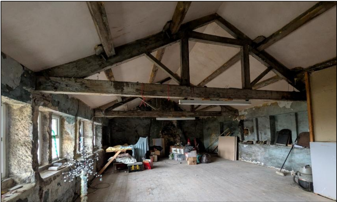
Plate 10. Image of roof space taken by third party, prior to vaulting, showing spray-foam insulation on underside of roof slates
