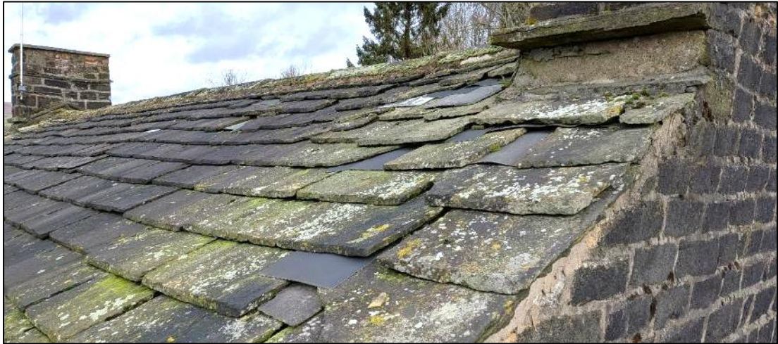
Plate 5. Inspecting gaps between stone slates on the mid-pitch
