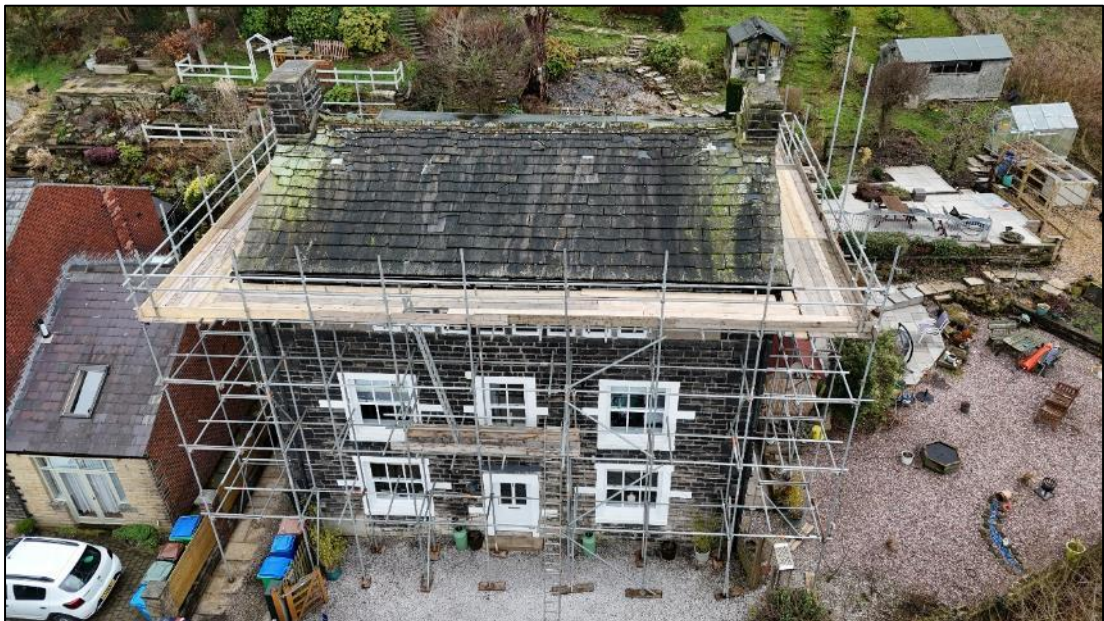
Plate 1. Façade – southwest elevation
