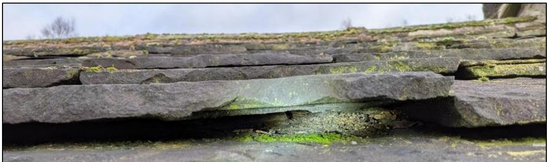
Plate 6. Larger gap between slates leading to void accessed by jackdaw, above northwest gable
