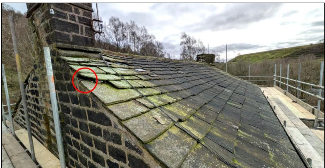
Plate 6. Larger gap between slates leading to void accessed by jackdaw, above northwest gable
