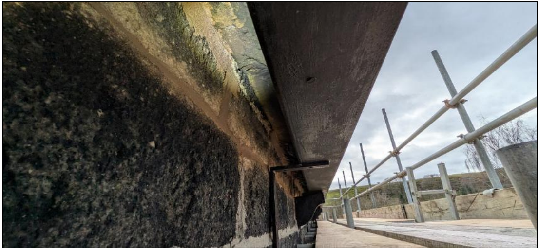
Plate 8. Gap between fascia board and wall on extension
