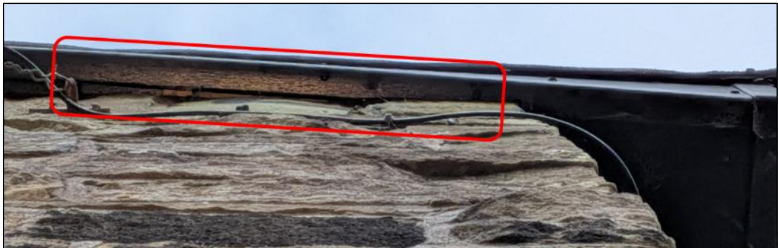
Plate 8. Gap between fascia board and wall on extension
