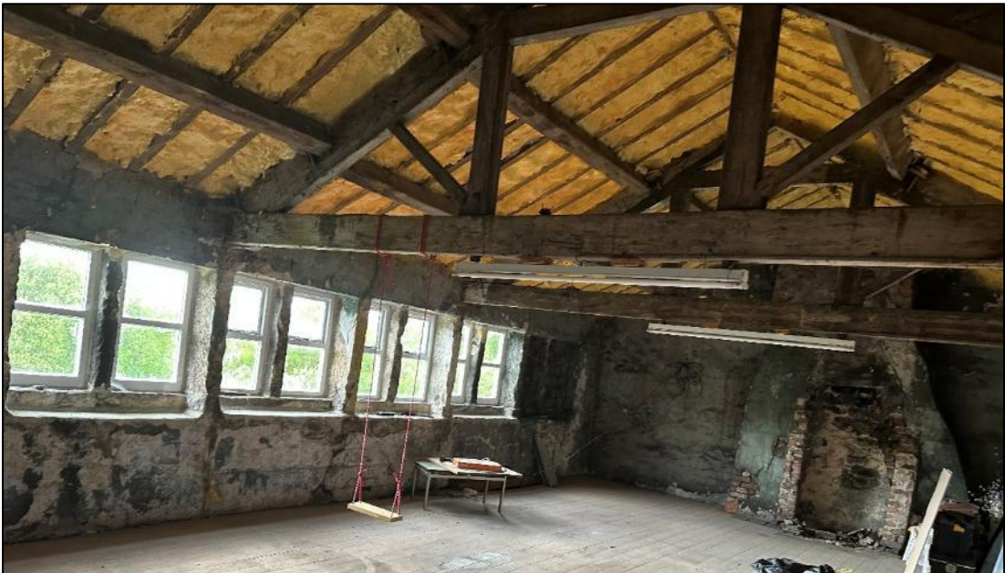
Plate 10. Image of roof space taken by third party, prior to vaulting, showing spray-foam insulation on underside of roof slates
