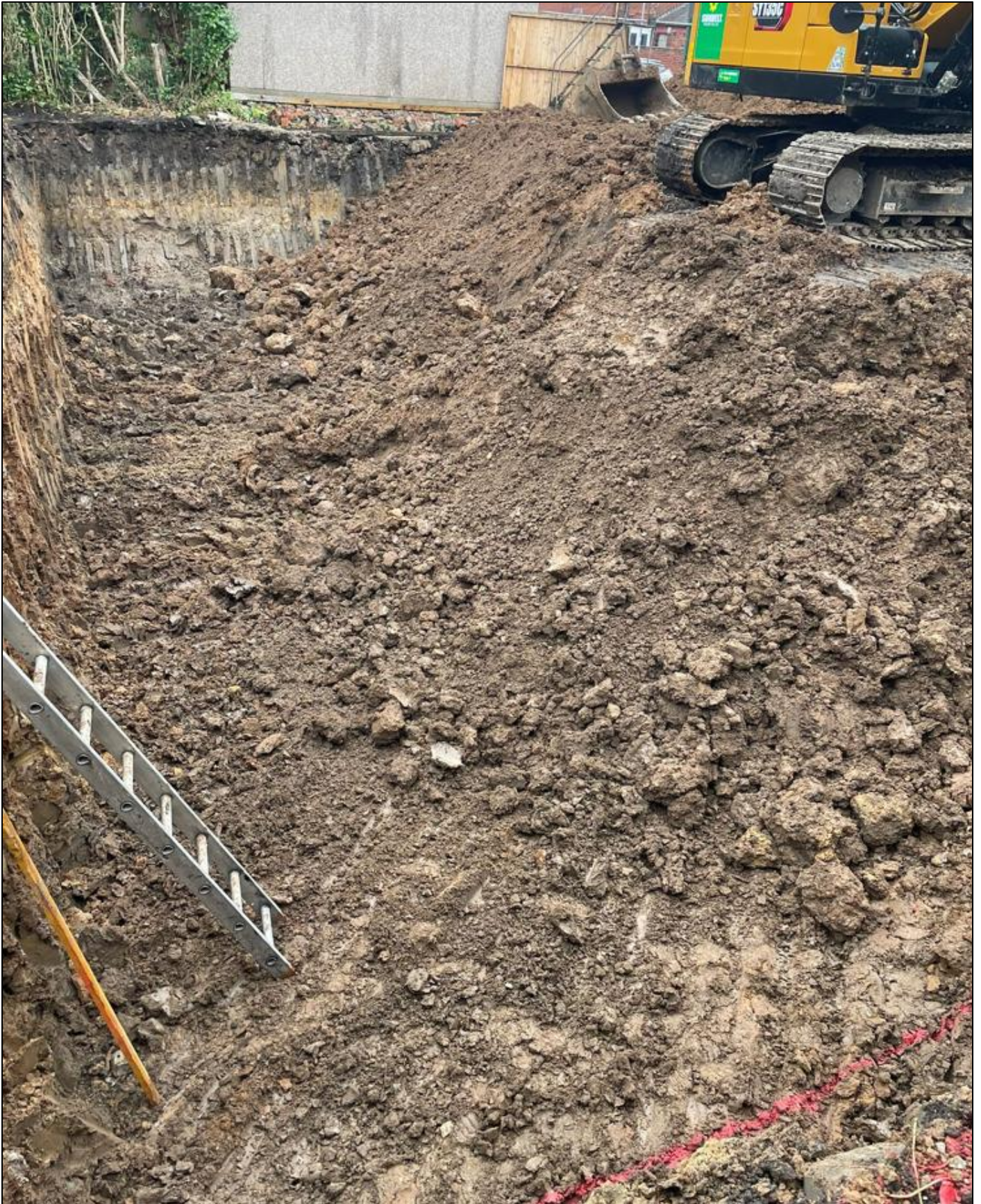
Site dig to approx 4m.
