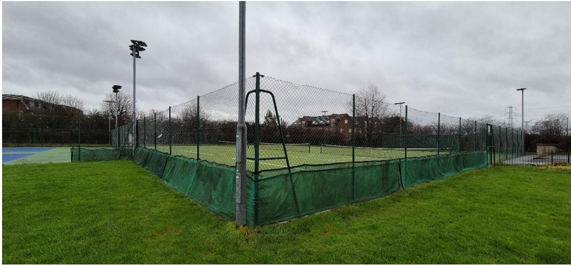
Existing Tennis Courts & Associated Lighting
